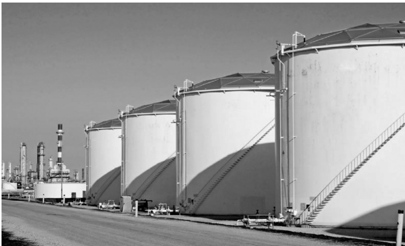
Figure 4.42 Tank farm in summer 2015. (Courtesy of Keller Group plc, London, UK.)
