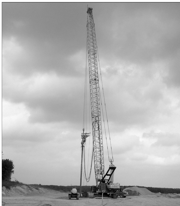
Figure 4.5 Crane-hung dry bottom feed system for deep stone columns (S-Alpha system). (Courtesy of Keller Group plc, London, UK.)
