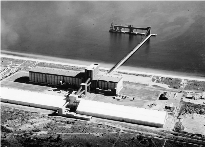
Figure 2.16 Areal view of the Grain Terminal at Kwinana, Western Australia. (Courtesy of Keller Group plc, London, UK.)
