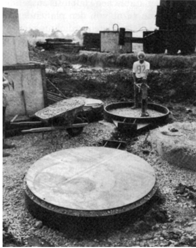
Figure 2.17 Preparation of a horizontal load test on vibro stone columns. (Courtesy of Keller Group plc, London, UK.)
