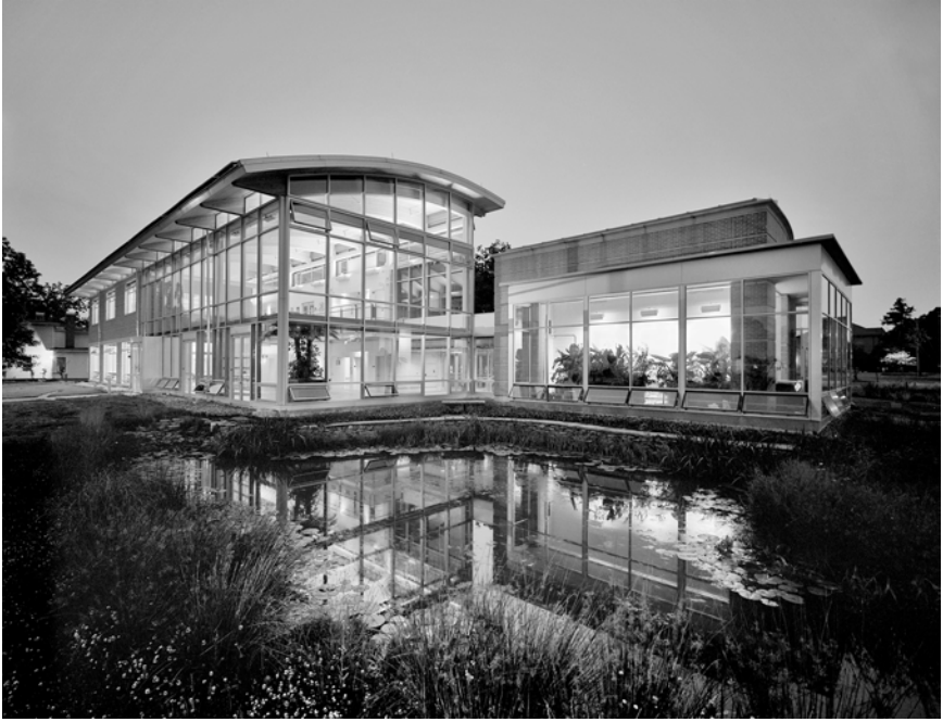
The Adam J. Lewis Center for Environmental Studies at Oberlin College, with exterior clad in aluminum. Courtesy Barney Taxel
