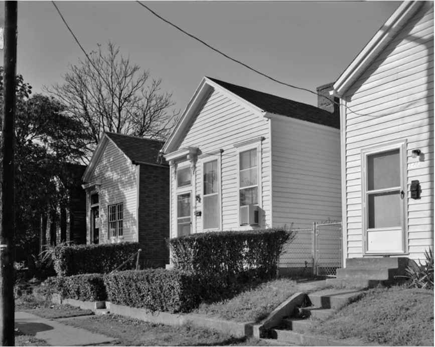
550 South 20th Street (house), Louisville, Jefferson County, KY, 1982. Aluminum siding, screen doors, and fences became common features of American vernacular architecture in the postwar era. Photograph by D. Mitchell, Historic American Buildings Survey, Library of Congress (HABS KY-190)
