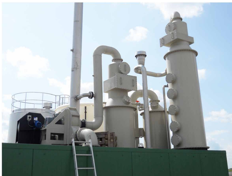
Figure 11. Ammonia stripping plant located in an agricultural biogas plant in Brescia, Italy - CRPA, 2015
