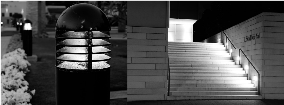
Fig. 22: Bollard lighting, recessed luminaires and illuminated stairs in the public domain
