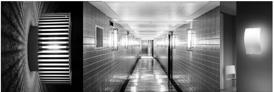
Fig. 24: Examples of wall lamps
