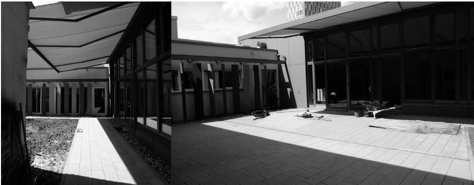
Fig. 12: Canopies designed to shade the window elements
