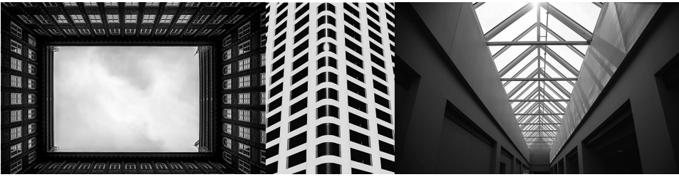
Fig. 7: The fenestration in the inner courtyard, the corner of the building, and the skylight
