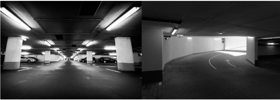
Fig. 29: Examples of lighting for underground car parks and multi-story car parks
