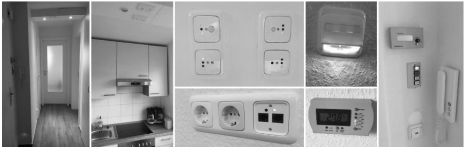
Figure 1. Apartment equipped with BASIS bus system (f.l.t.r): corridor with nightlights, kitchen with sensor array at ceiling, sensor array (PIR, VOC, temperature, brightness), controlled power sockets with smart meter, night light, heater control, text display at entrance door.
