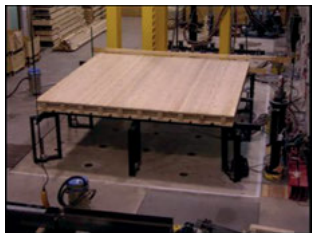
Fig. 6.12: Suspended floor of dimensions 4 m × 4 m × 0.22 m built exclusively by rotational dowel welding.
