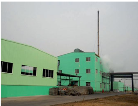
Fig. 5.50: Boiler house of the Excelic Food Technology Company.
