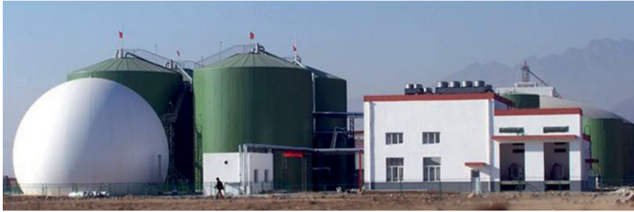
Fig. 4.43: Beijing, DE Qing Source's 2 MW cogeneration biogas engineering of fowl manure.
