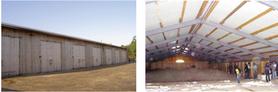
Fig. 4.16: External and internal structures of carport dry fermentation digester.
