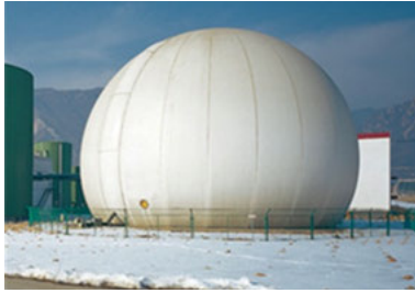
Fig. 4.25: Double-membrane dry gas storage cabinet structure.
