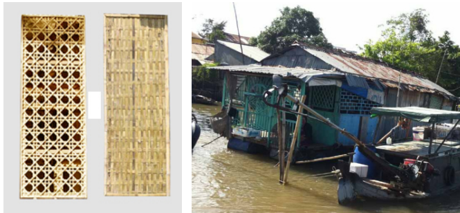
Fig. 11 The façade of floating houses are made of wickerwork, latticework, and reed weaves
