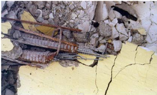
Corrosion of reinforcing bars
