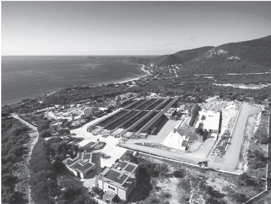
Figure 7.35: MYRTE installation (University of Corsica).
