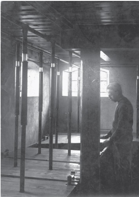
Figure 3.2: Electrolysers used by Poul la Cour (Poul la Cour Museum, Vejen).
