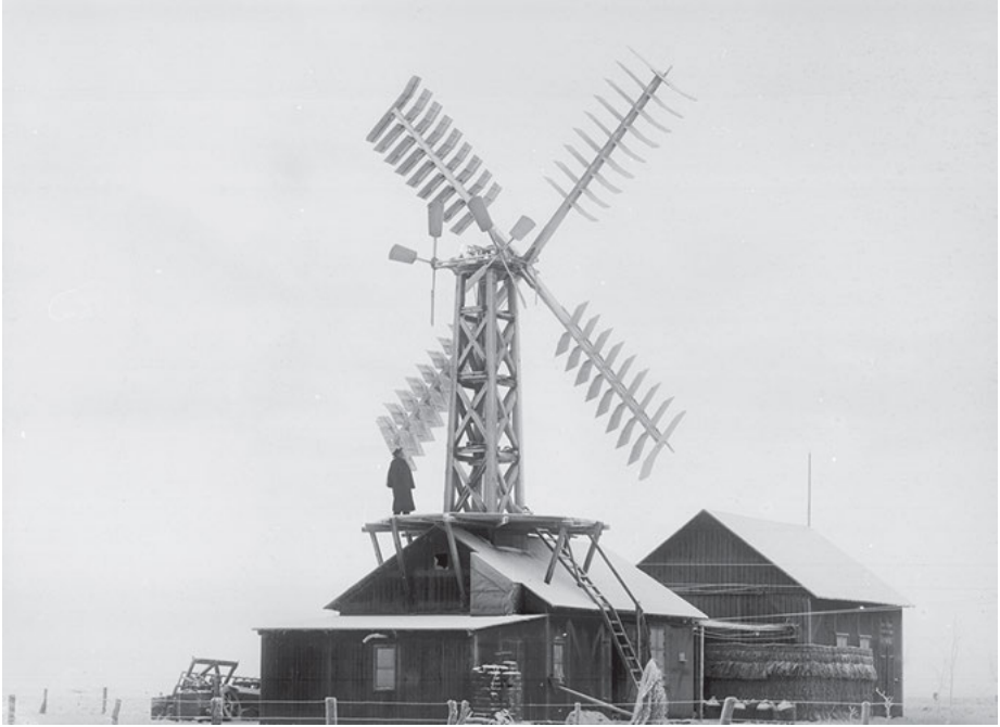
Figure 3.1: Windmill transformed into a wind turbine by Poul la Cour (Poul la Cour Museum/Vejen).
