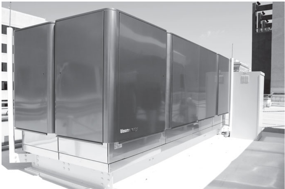
Figure 5.32: A 100 kW SOFC fuel cell module (Bloom Energy).
