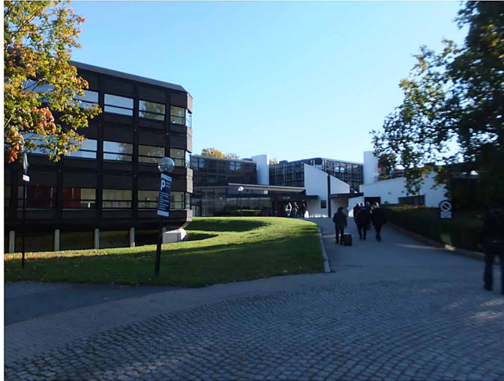
Figure 1. Kjørbo Building: View from the main path Powerhouse Kjørbo, 2016.
