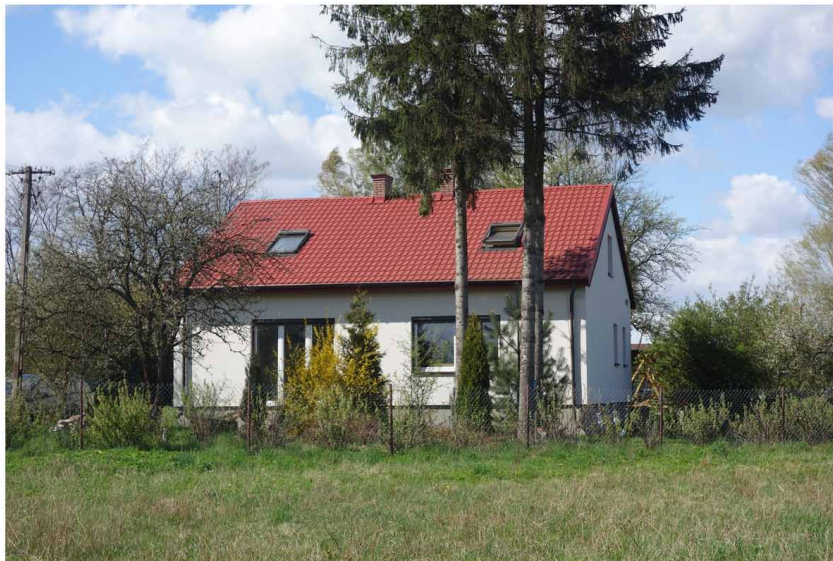
Figure 8. Building after the energy retrofit KAPE SA, 2016.
