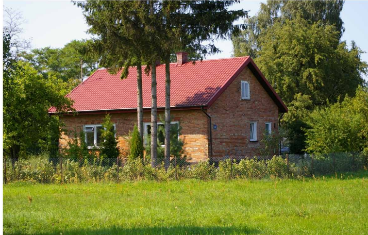
Figure 1. Photograph of the house before the energy retrofit KAPE SA, 2016.
