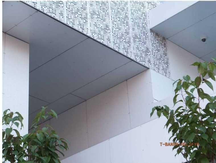
Figure 7. Detail of retrofitted façade perforated cladding, Fredrik Selmers vei 4 KodnZEB, 2015.
