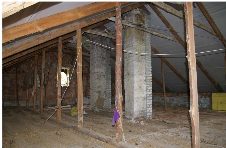
Figure 4. Visible roof construction and steel joist ceiling above the ground floor © Copyright KAPE SA, 2016.
