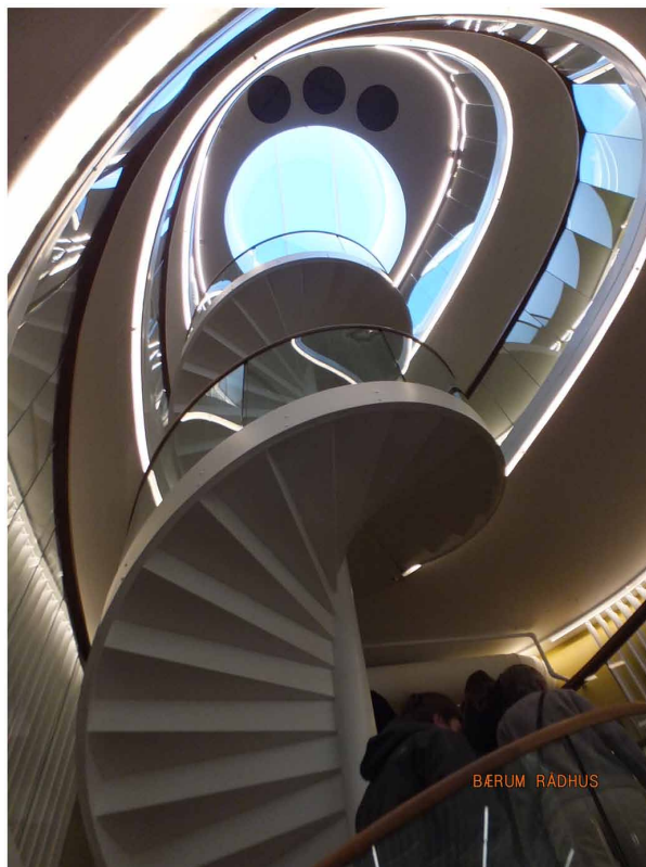
Figure 2. View of the spiral staircase used as extraction air duct, but also as possible means of communication between floors Powerhouse Kjørbo, 2016.
