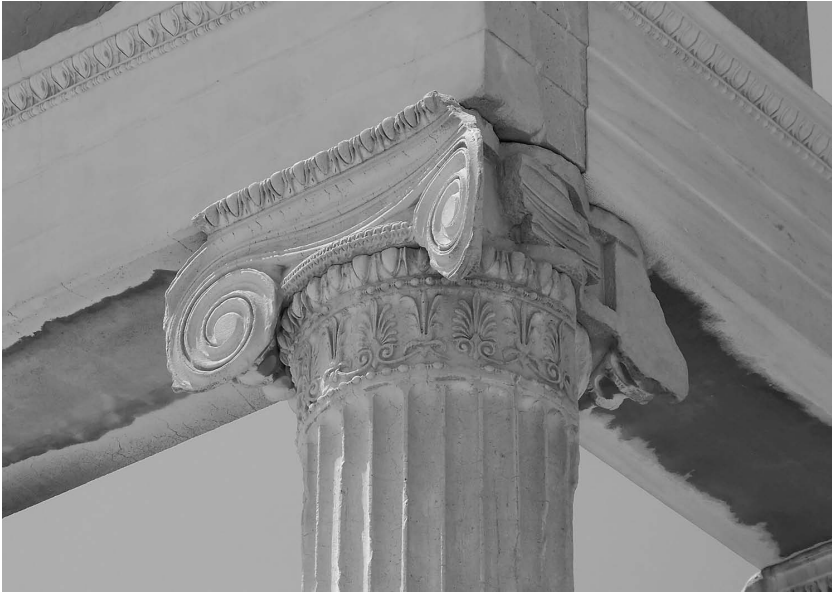
Figure 4.9. Erechtheion, Athens (421–406 BCE): Capital and architrave from the east façade. Photo by Guillaume Piolle.
