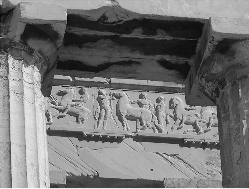
Figure 6.5. The Parthenon, west façade: detail showing Doric capitals and Ionic frieze with Doric guttae underneath. Photo by Athinaios.
