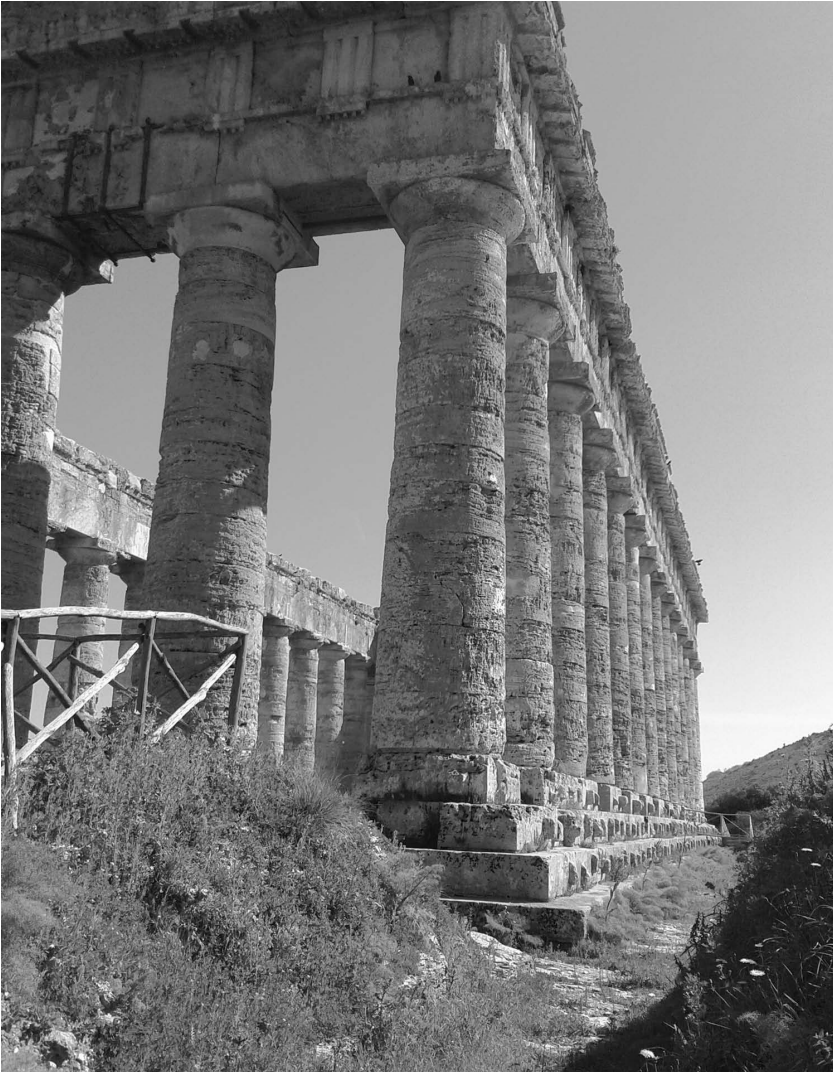
Figure 5.9. The Temple at Segesta: view from the southwest corner, showing curvature. Author's photo.
