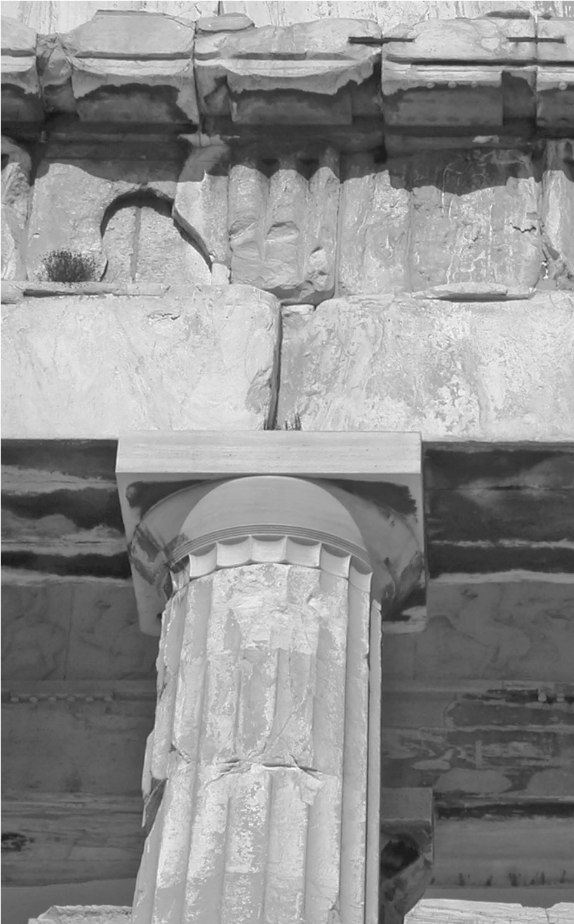
Figure 4.5. The Parthenon: column capital and entablature, west façade. Source: Creative Commons.
