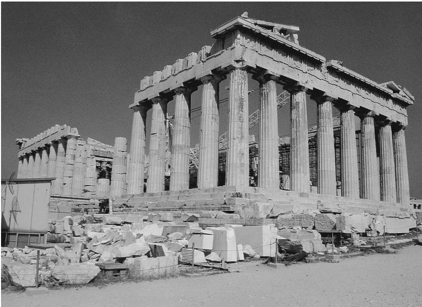
Figure 4.2. The Parthenon: view from the southeast. Photo by Peter van der Sluijs.
