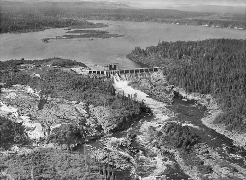
In the 1930s, the Chicago Tribune Company built a dam on the Outardes River to fulfill one of the conditions of its North Shore forest concession and to generate power for its operations in the region. This aerial photo shows the operational dam in 1937. Vol. 25198, folder Outardes (1 of 2), QOPC, LAC. Used with permission.
