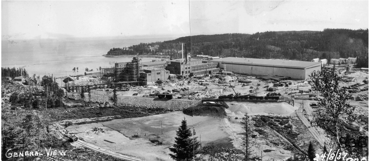
By late August 1937, the Tribune Company had made significant progress on its Baie Comeau mill construction. Vol. 25178, Scrapbook 1934–41, QOPC, LAC. Used with permission.
