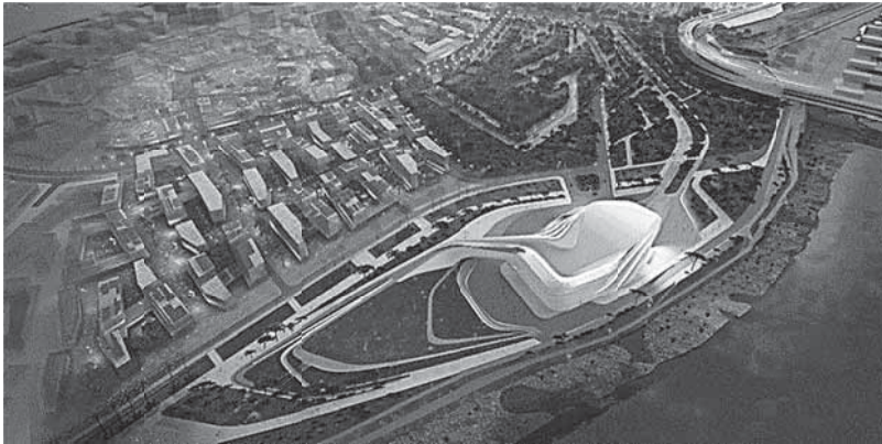
Figure 01.5 Grand Théâtre de Rabat. (Image courtesy of Zaha Hadid Architects at www.zaha-hadid.com )
