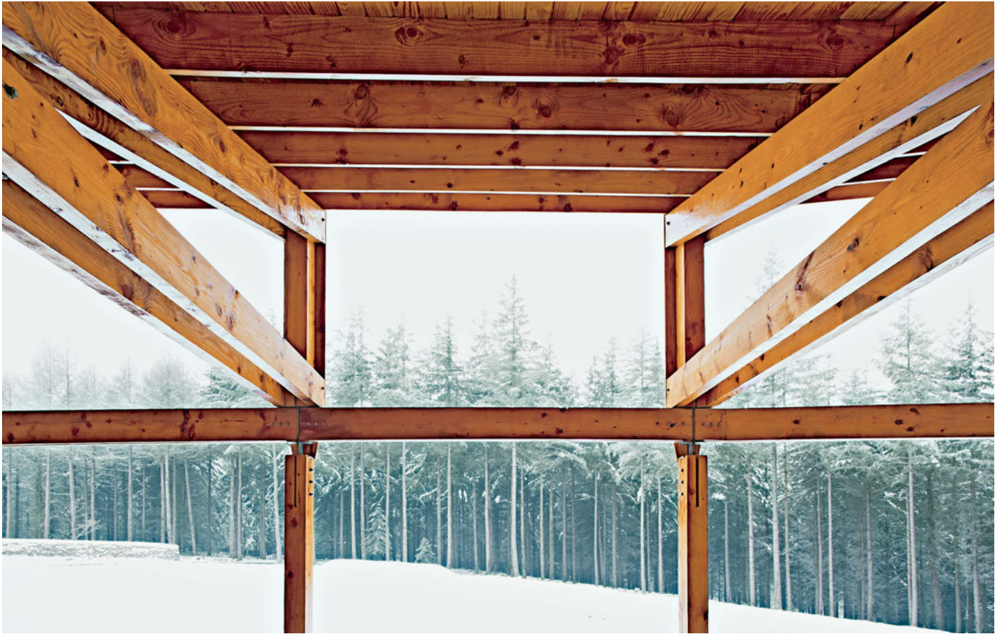
The wood-frame structure is built using sustainably harvested wood from local forests; the wood siding is left untreated and exposed to the elements.
