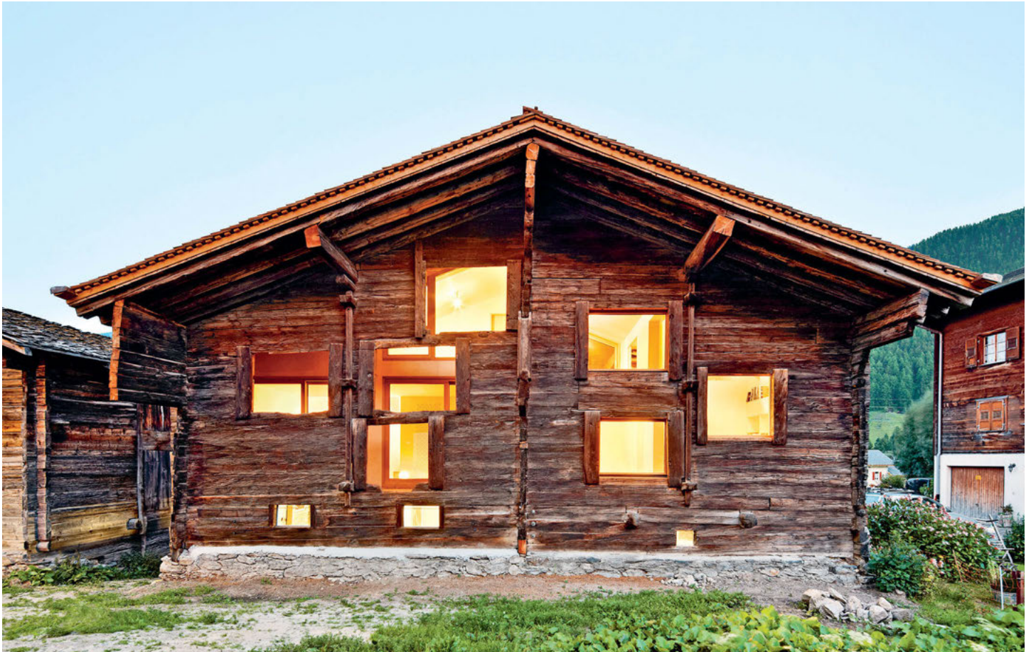
To preserve the historic log structure in its original state, a timber "insert" was integrated into the existing structure.
