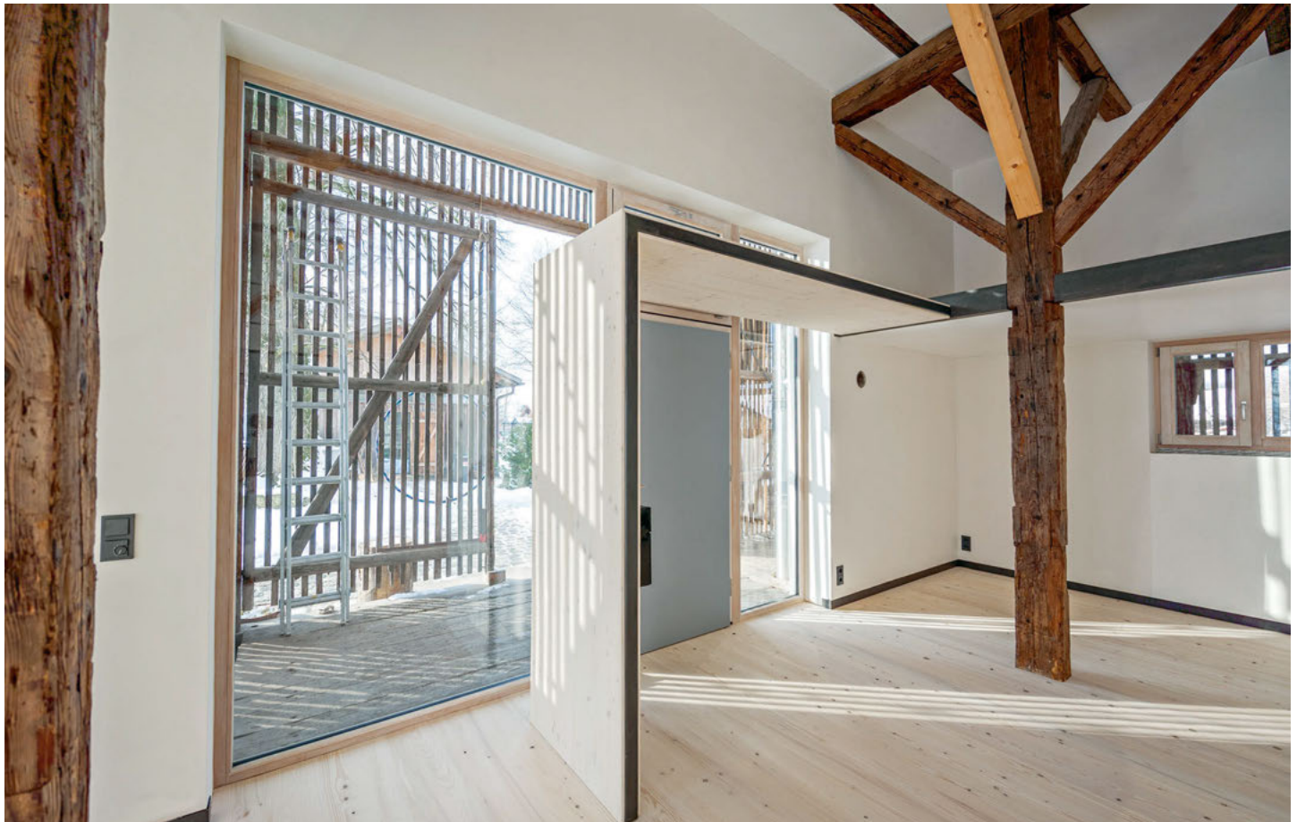
Once the peat barn had been rebuilt, a structure was set off-center within the old load-bearing frame of the barn according to the house-within-a-house principle.
