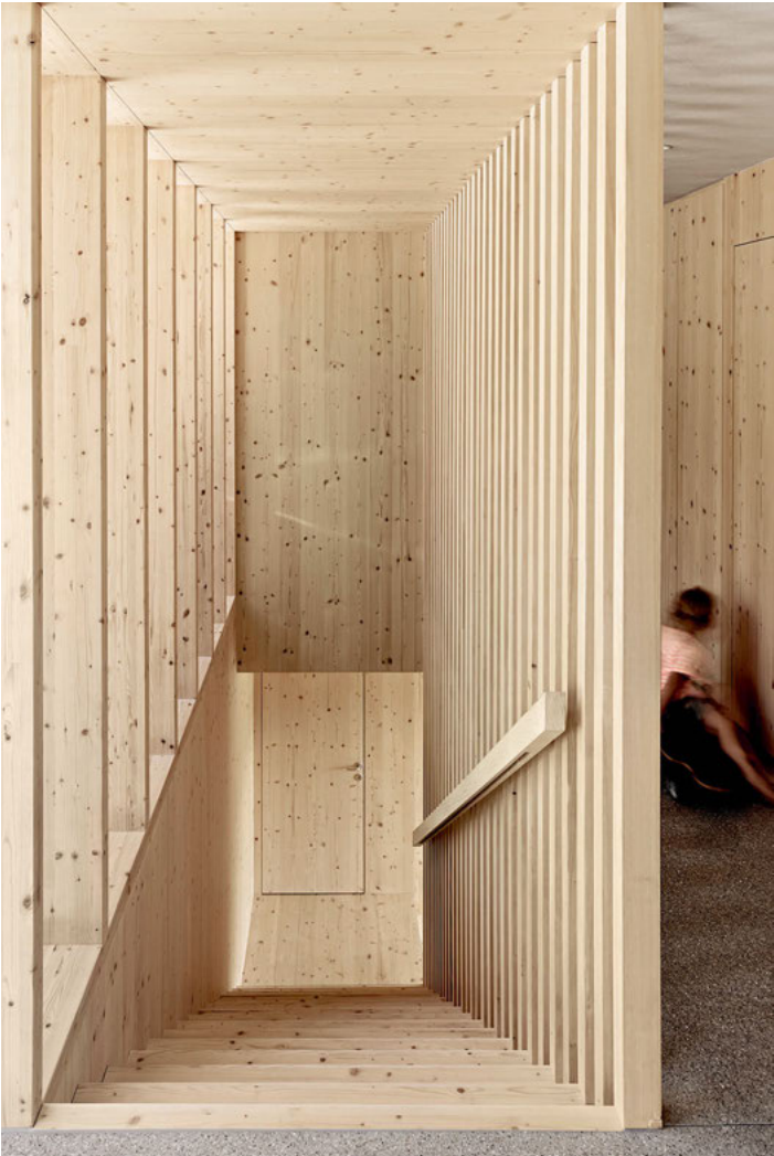
Spruce from the client's own forest was used for the roughly sawn and soaped wood flooring as well as for built-in furnishings, staircase, and wall cabinets.
