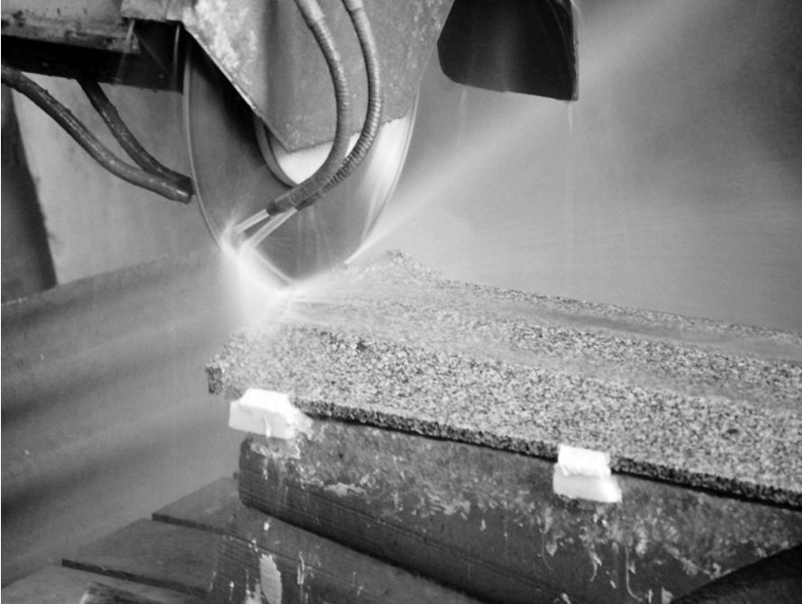
Figure 2.5 Robot saw cutting (eight-sided central nave column).
