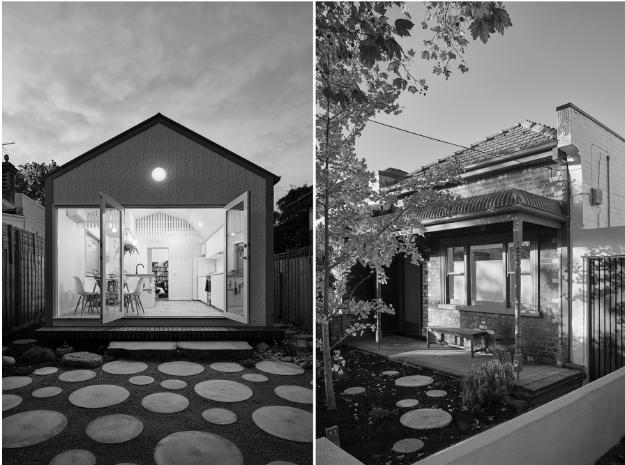
Figure 5.1 Avery Green from the front and back after 2015–16 alterations.
