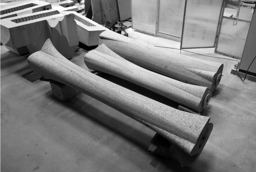
Figure 2.12 Columns for the Sagrada Família basilica Passion façade awaiting delivery to site, ready to incorporate into the narthex. No additional work is required on site in the twenty-first century, whereas in a previous generation the construction site was also the masons' yard.
