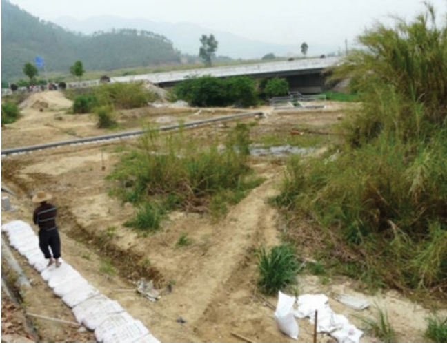
Figure 6.7: Before the construction.
