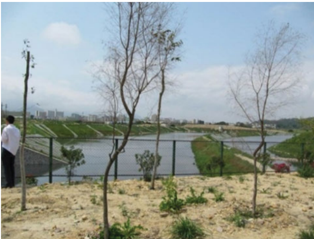
Figure 6.17: The status of depth treatment 1.
