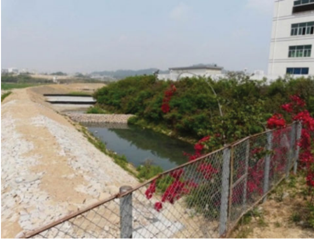
Figure 6.18: The status of depth treatment 2.
