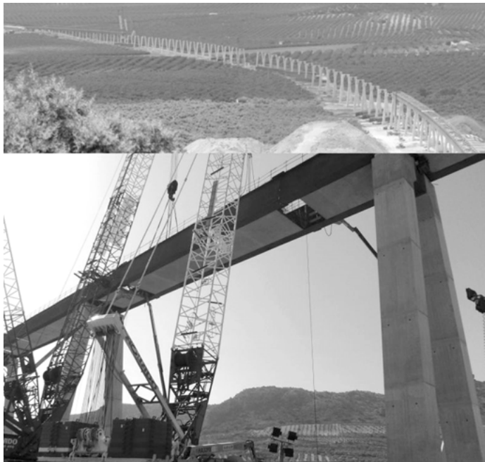
Fig. 11: Archidona (Spain) viaduct: continuous composite twin-girder bridge with upper and lower concrete decks. Image courtesy of Alejandro Castillo Linares ( http://www.acl-estructuras.com ).
