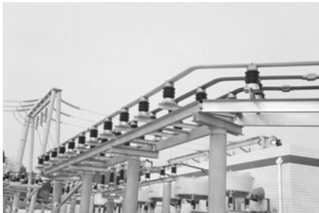
Fig. 1: The 35 kV busbar bridge for analysis. There are three phase conductors on the bridge. The cross-section of the rectangular conductors is 125 mm × 10 mm. The conductors are equidistant with a distance of 0.4 m and loaded with symmetry currents of 1039 A.
