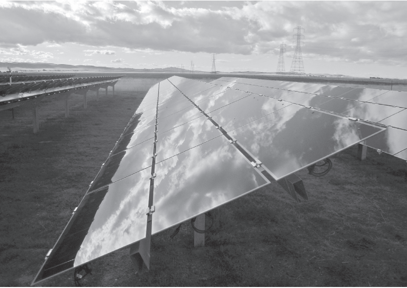
FIGURE 15. The Topaz Solar Farm in San Luis Obispo County, California, uses CdTe thin-film photovoltaic modules.
