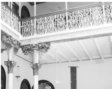
Figure 6: Victorian Scottish cast-iron columns and railings.
