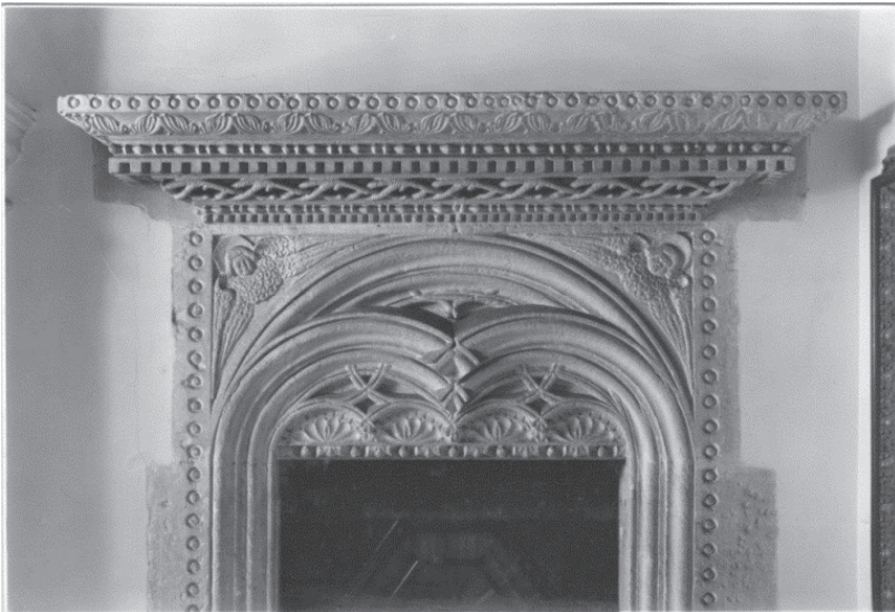
2.2 Detail of window-frames at Wawel Castle by permission of the Instytut Historii Sztuki, Jagiellonian University, Kraków
