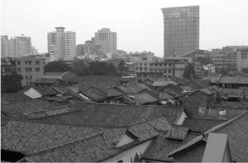
Figure 9.6 Restored courtyard houses, Wenming Street
