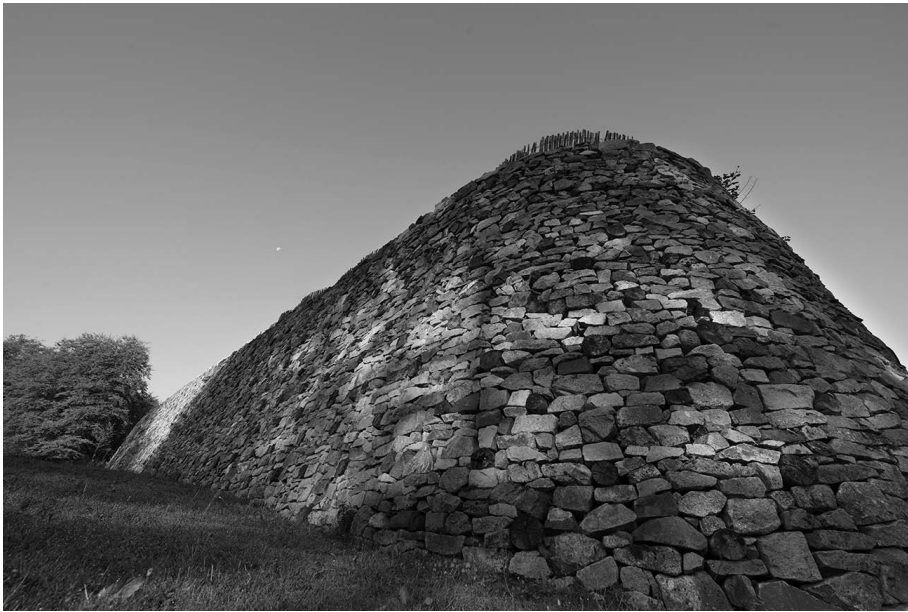
FIGURE 4.9. Bibracte -Mont Beuvray. Reconstruction of the impressive murus gallicus of the Porte du Rebout (after Rieckhoff 2014).
