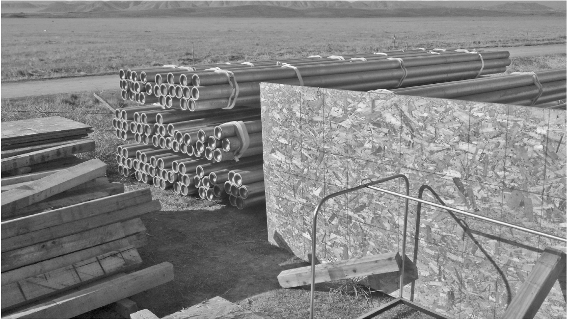
Figure 8.2 Example of piles plugged and barricaded to minimize use by wildlife. H. T. Harvey & Associates.
