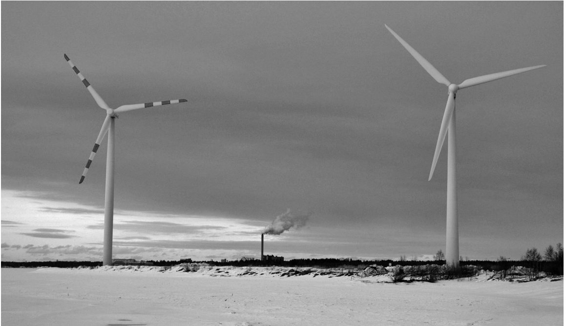
Figure 5.5 Painting turbine blades to increase visibility (left) is a proposed mitigation technique to reduce or eliminate bird collisions with wind turbines. Thus far, empirical evidence is lacking to support this as an effective mitigation technique. Photo credit: Imwindpower.com.
