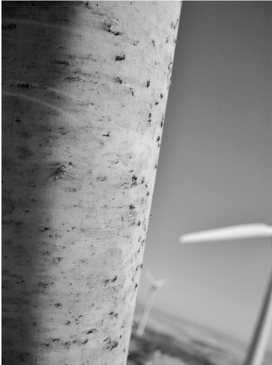
Figure 7.3 Insect collisions with turbine blades can be substantial and reduce power generation. Used with permission from BladeCleaning.com.
