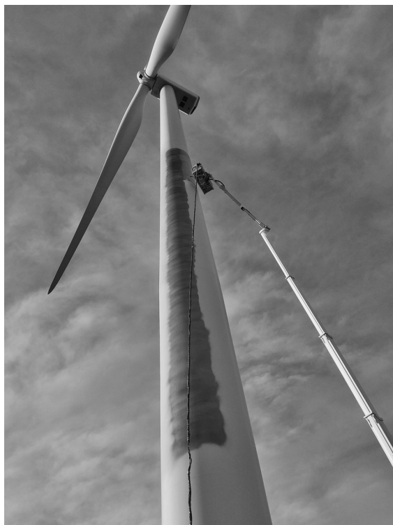
Figure 11.1 Texture coating being applied to the monopole of a wind turbine at the Wolf Ridge wind energy facility, Texas, US; this textured coating may help mitigate bat mortality at wind energy facilities by deterring bats from interacting with smooth tower surfaces. Photo credit: Amanda Hale.
