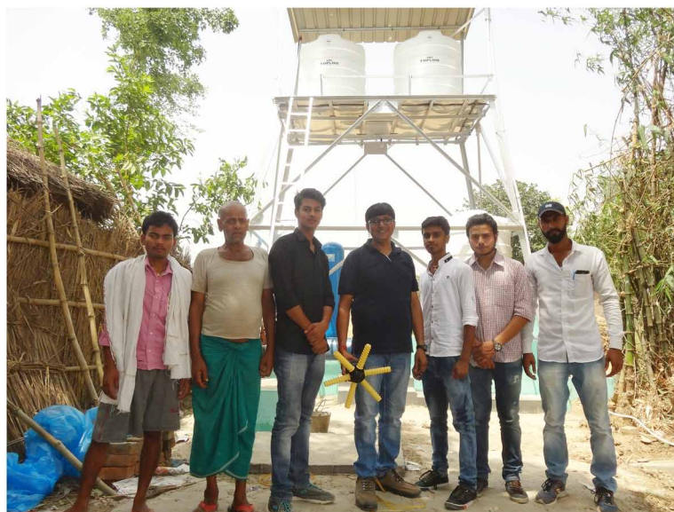
Figure 13. Installation of arsenic filter
