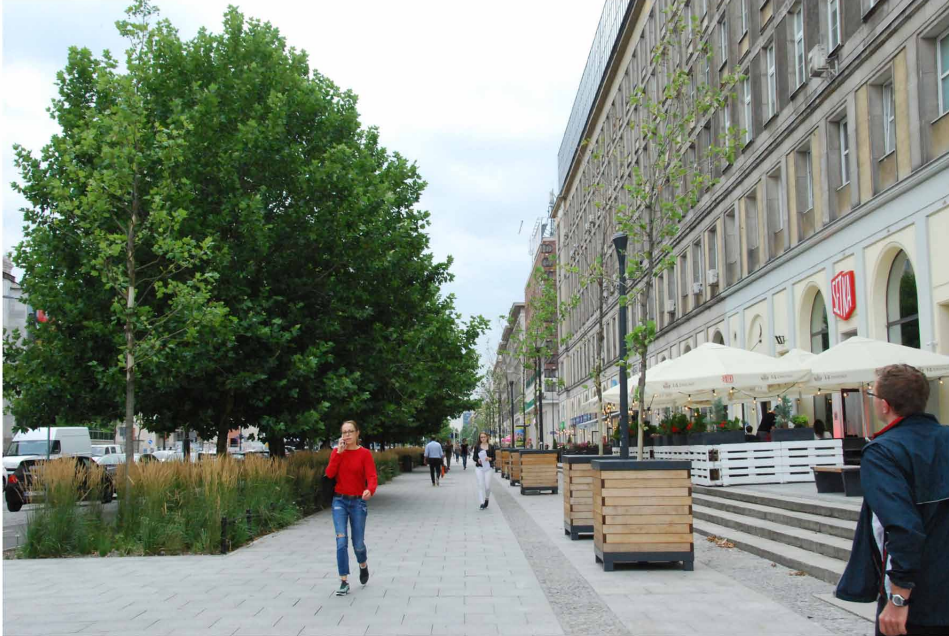
Figure 14. A fragment of the communication route Świętokrzyska Street after reconstruction, introduction of greenery, bicycle paths and narrowing of the carriageway. The investment has been widely praised (photo by the author, 2018)
