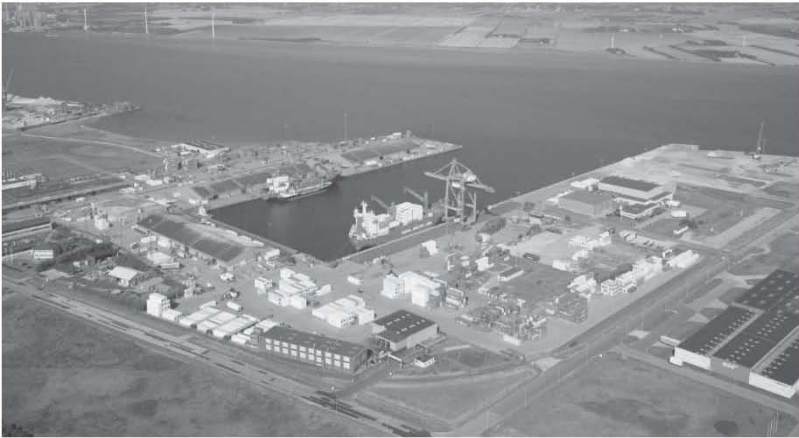
Fig. 9.9. Port of Aalborg, Denmark
