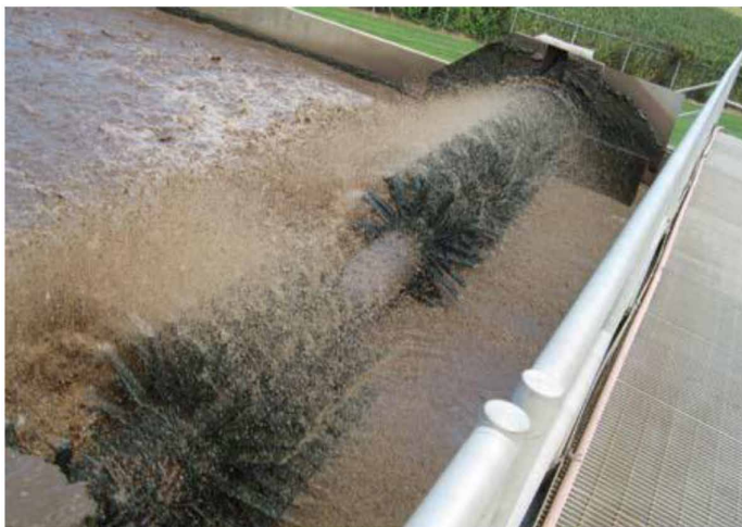
Figure 6. Mechanical rotor aerators
