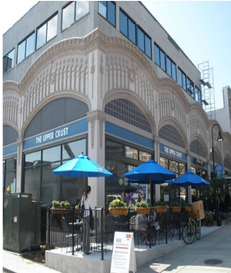
Figure 19. Boston University's geothermal building (Lebovits, 2010)
