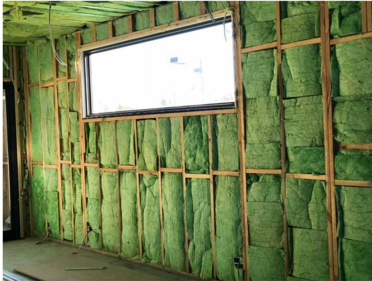
Figure 4. A wall with green insulation
