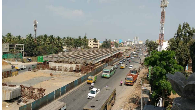
Figure 1. Construction of flyover bridge
