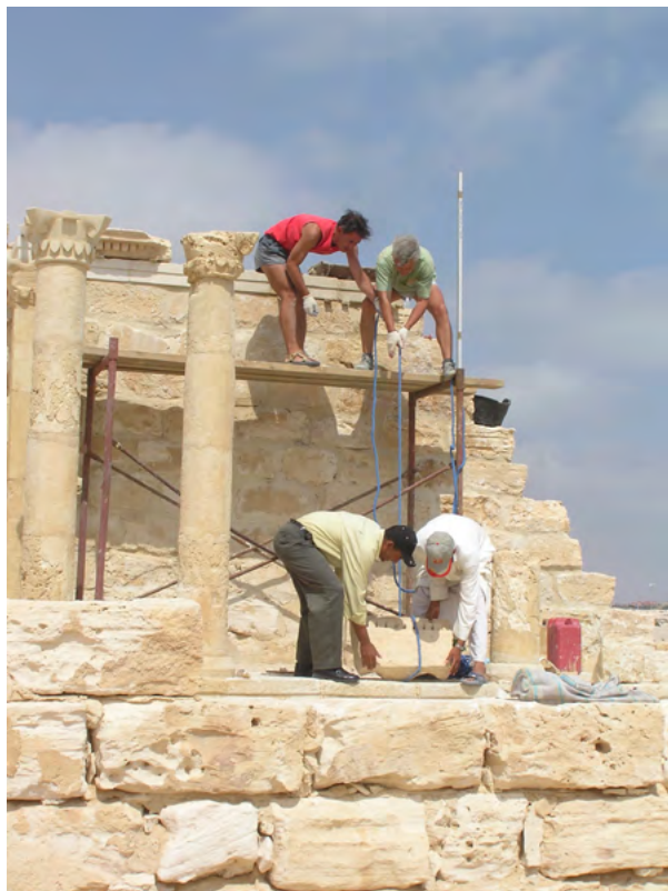
Figure 7. Assembly of elements of a cornice crowning the commemorative monument to Commodus (Photo M. Mrozek-Wysocka)
