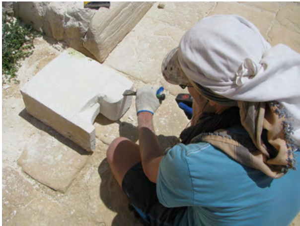
Figure 5. Making a copy of a bench leg (Photo W. Grzegorek)
