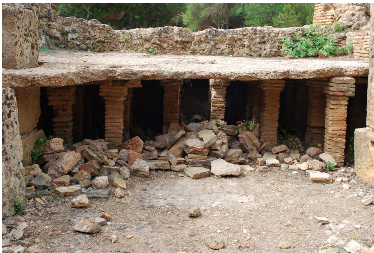
Figure 6. Tipasa. View of the hypocaustum in Small Baths (Photo M. Czapski)
