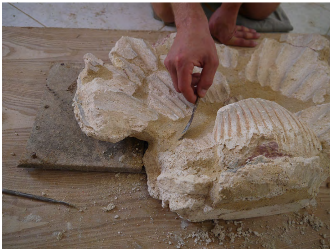
Figure 17. Shell of lime mortar. Conservation work. Filling in with mineral mortar (Photo M. Koczorowska)
