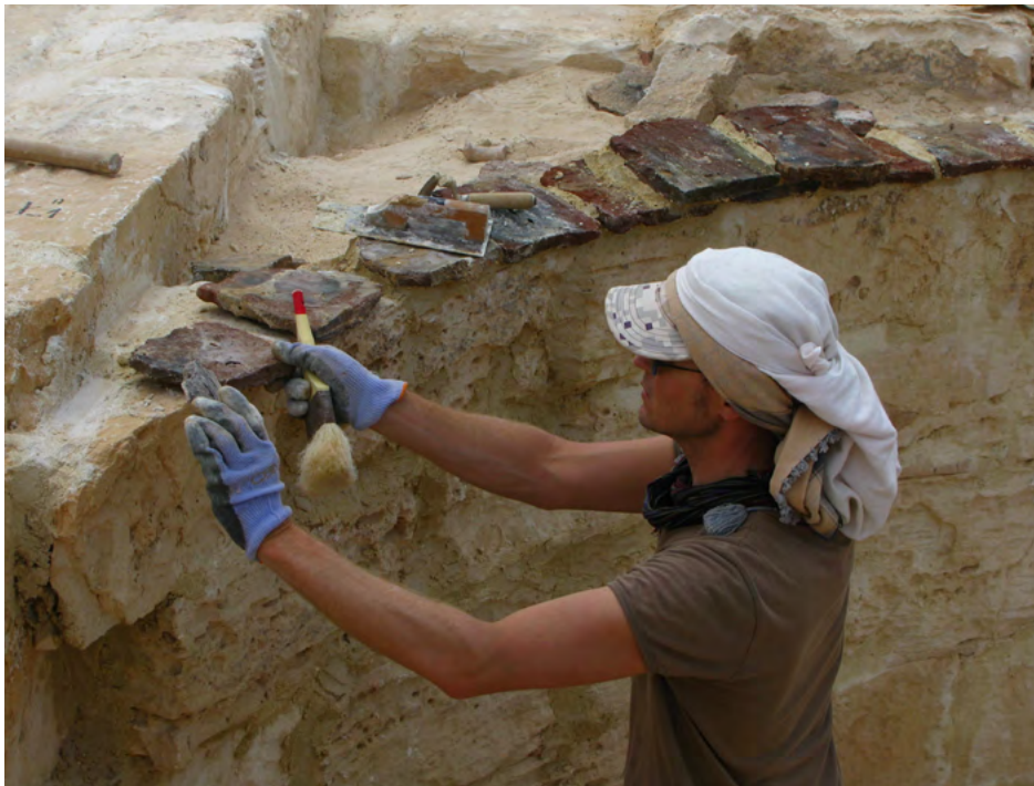
Figure 10. Tholos. Bricklaying during the reconstruction of the dome's base (Photo W. Grzegorek)
