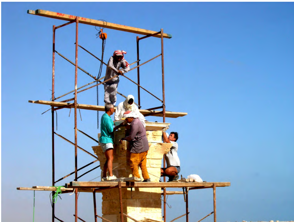
Figure 4. Work on the scaffolding on the anastylosis of a part of tomb T1K above the capital (Photo S. Medeksza)
