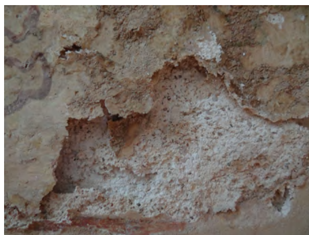
Figures 10, 11 and 12. In the photos, the condition of the item after re-entering the storerooms in 2013 is visible. In close-ups, the results of salt migration are visible: the detachment and destruction of the paint layer together with the mortar ( Photos M. Koczorowska )
