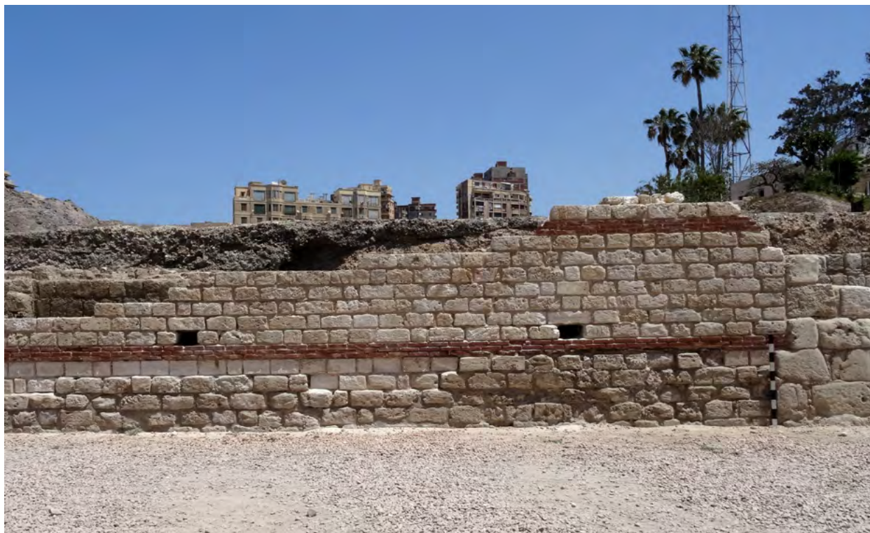
Figure 14. Portico back wall, visible putlogs. Scale length: 1 m (Photo G. Majcherek ©PCMA)
