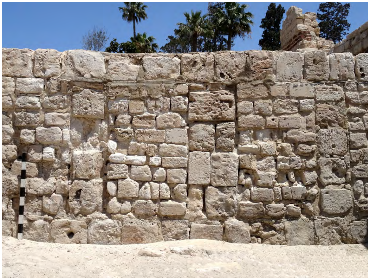
Figure 13. Wall built in the opus africanum technique. Scale length: 1 m (Photo G. Majcherek ©PCMA)
