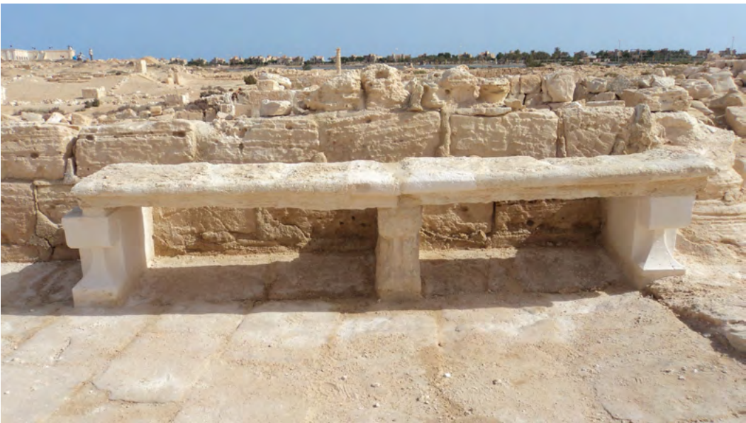
Figure 4. Filling in a gap in a half round of a seat with a cover (Photo W. Grzegorek)
