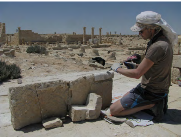
Figure 4. Filling in a gap in a half round of a seat with a cover (Photo W. Grzegorek)
