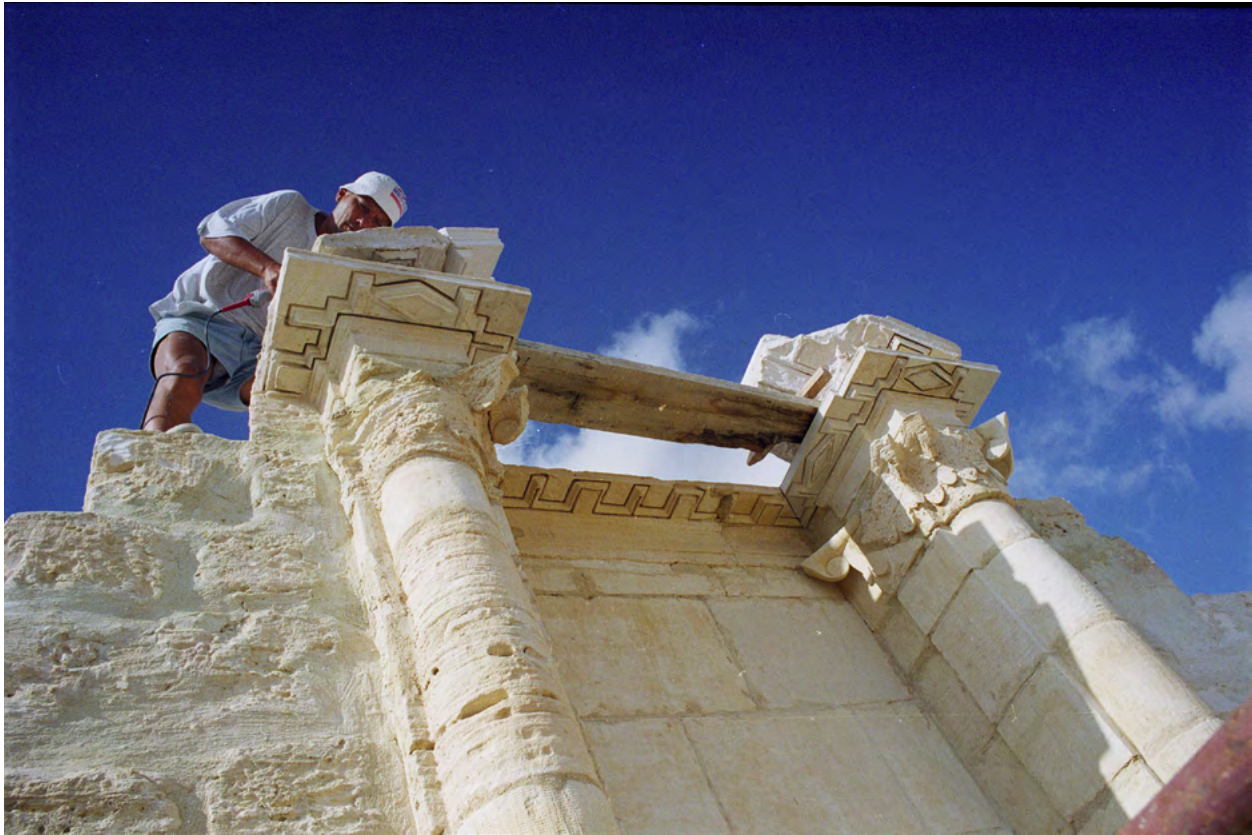
Figure 10. Assembly of elements of a pediment in the aedicula in house H21'N' (Photo R. Czerner)
