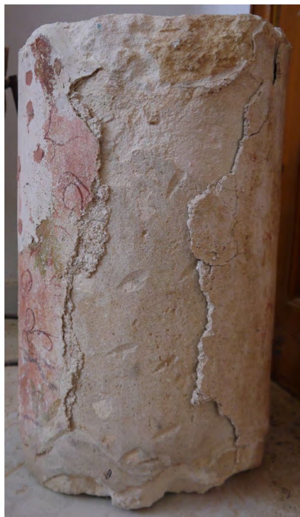
Figure 13. Photo before conservation. Detachments of the mortar layer are visible together with the paint layer (Photo M. Koczorowska)
