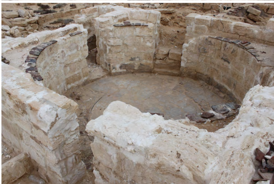
Figure 9. Tholos after conservation. Reconstructed base of a brick dome (Photo R. Czerner)
