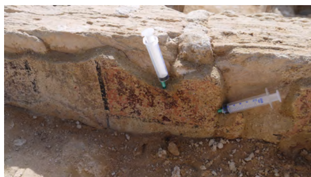
Figure 2. Photo with a fragment of a polychrome discovered at the site visible while protecting the item from detachment. The empty spaces between layers were filled in with synthetic hydraulic lime (Photo M. Koczorowska)
