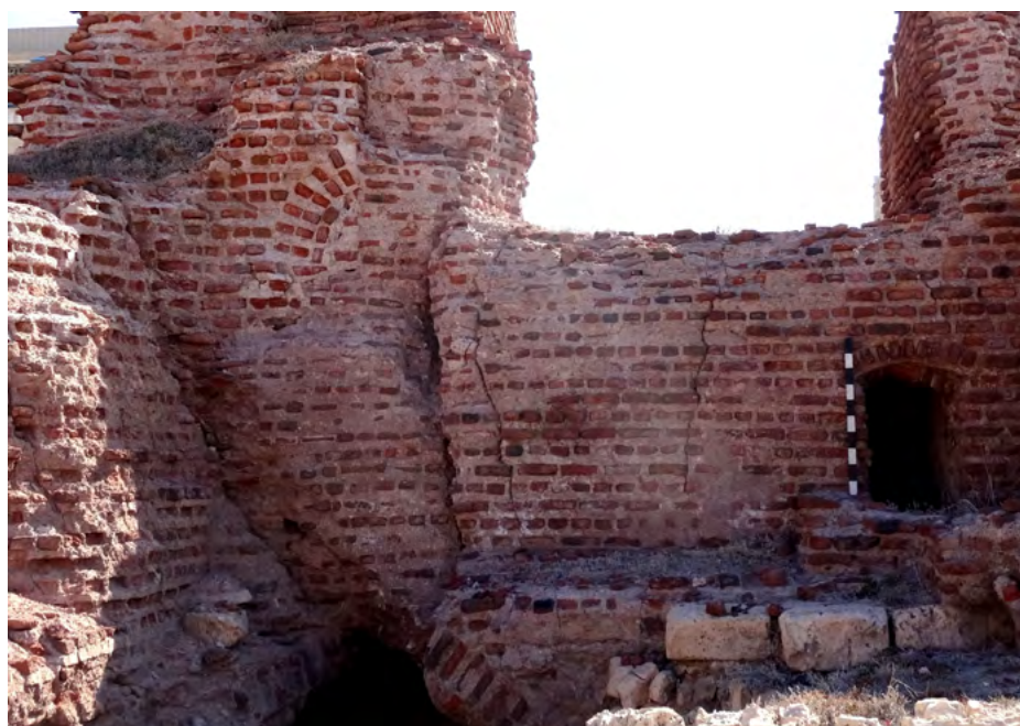
Figure 11. Damaged walls in the bathhouse, evidence for seismic destruction. Scale length: 1 m (Photo G. Majcherek ©PCMA)
