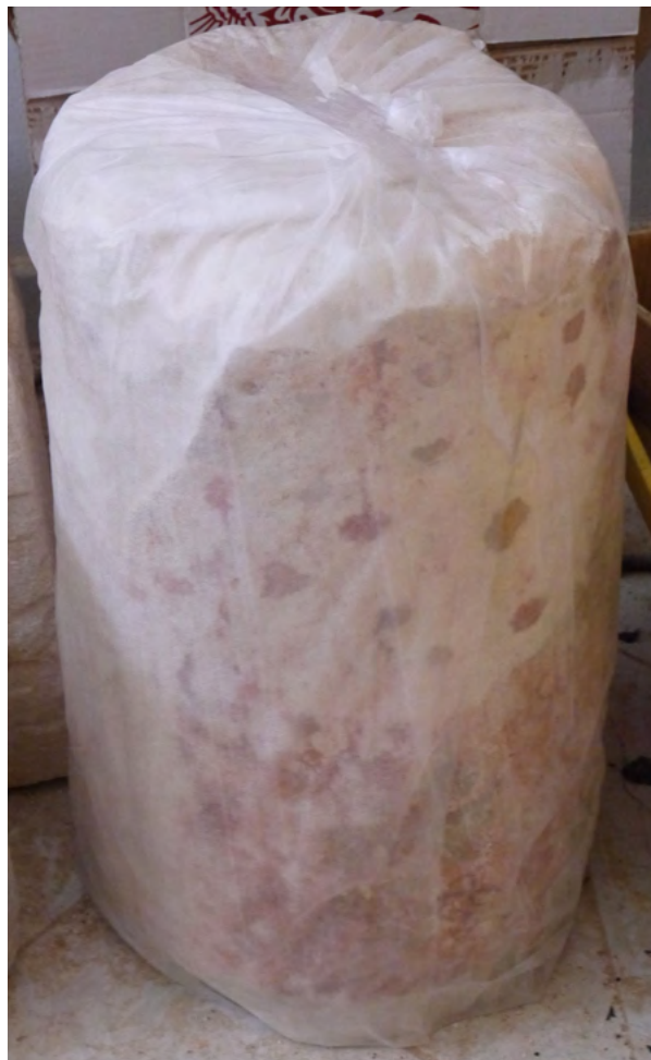
Figure 16. Column's shaft protected with interfacing (Photo M. Koczorowska)
