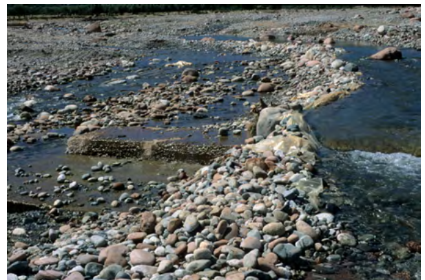
Figure 11. Diversion dam of the Tasultānt Qbīla sāqiya taking water from Ūrika wādī (Photo R. González Villaescusa).
