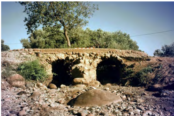
Figure 13. The medieval urban area overcame the obstacle of the Tasuṭānt Qbīla sāqiya thanks to two arches made of stone masonry and brick which nowadays, in the modern village, serve as a bridge for pedestrians and light vehicles (Photo P. Cressier).
