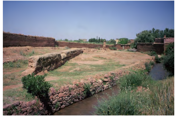
Figure 9. Remains of a medieval channel bypass sāqiya Tasultānt Qbīla, and the mill it supplied, in the town center of Aǧmāt Ūrika (Photo P. Cressier).
