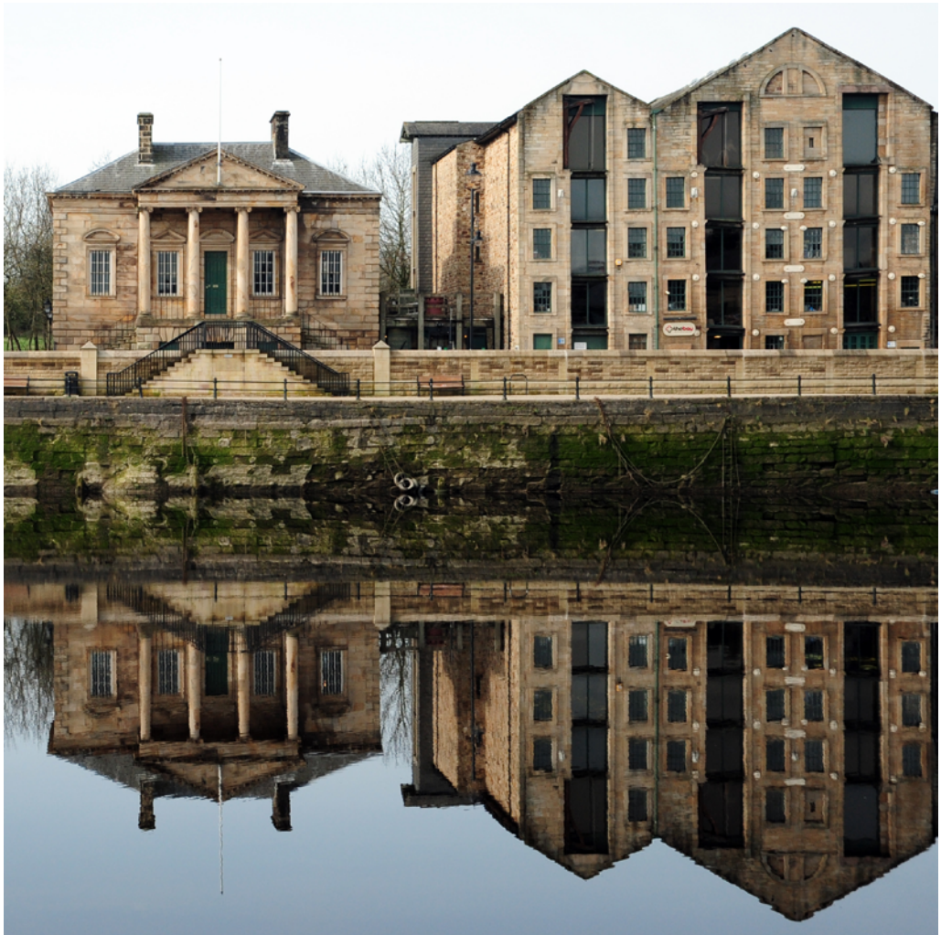
Figure 6. Eighteenth Century Custom House and Warehouses, Lancaster (Nisbet).
