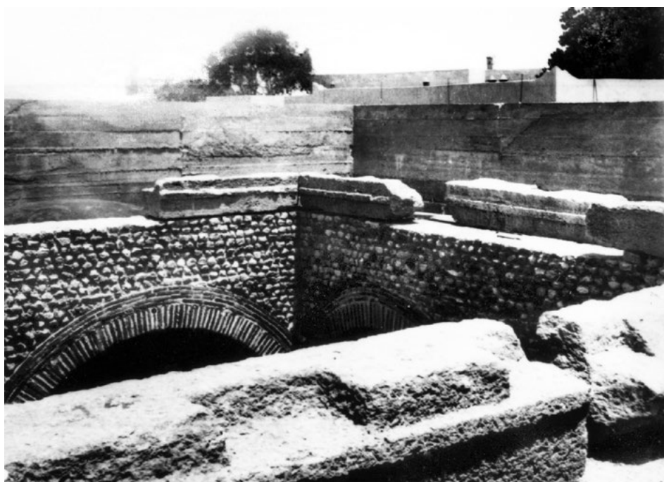
Figure 5: Cos, the latrine- nymphaeum during the reconstruction in 1938-1939. On the upper part of the inner front a series of prasinopetra blocks, clearly architrave-frieze elements, were mounted. On the rear they have recesses for the beams of a roof irrelevant to the latrine- nymphaeum (photo: L. Morricone, SAIA Archive, no. M934).
