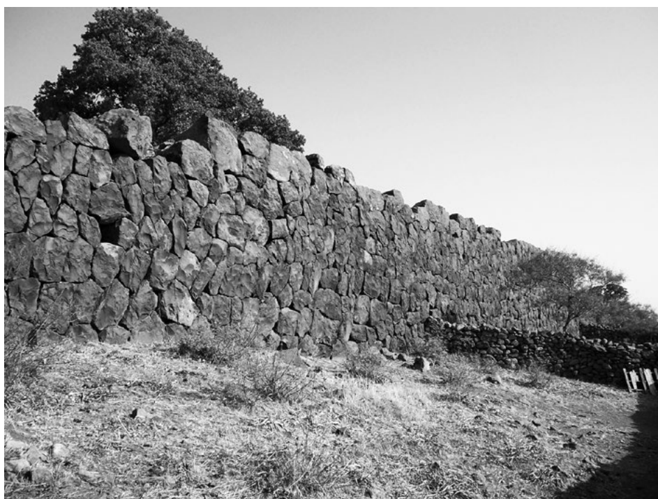
Figure 4. The Archaic (first half of the 6th century BC) terrace-wall in Apotheka, known as Kalochtistos (well-built) or Rodotoichos . The wall is the best preserved example of Lesbian masonry on the island of Lesbos (photo: © Copyright Hellenic Ministry of Culture and Sports, Ephorate of Antiquities of Lesbos).
