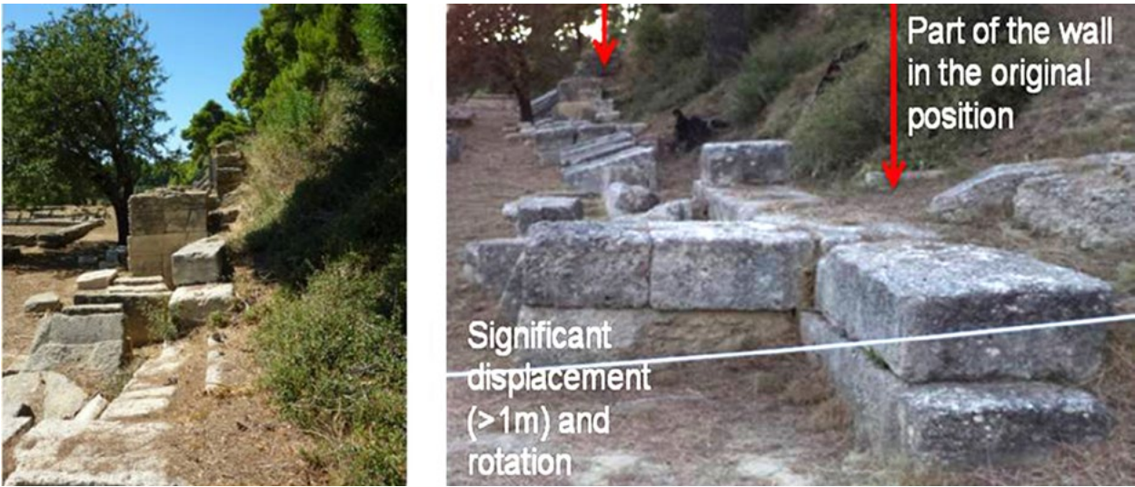
Figure 5: Collapse of east segment and horizontal displacement jump (photos: D. Egglezos).
