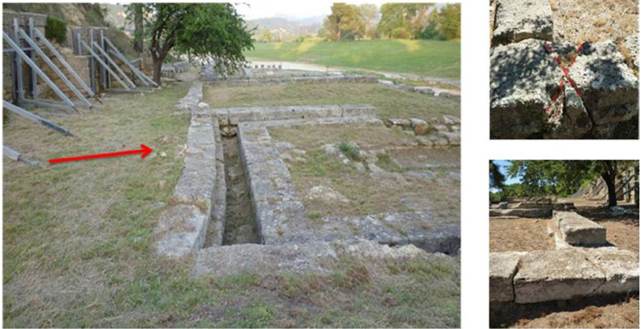
Figure 6: a) Horizontal displacement (0.05-0.25 m) of foundation blocks of north segment of easternmost Treasures (left), b) Characteristic shear fracture of the NE cornerstone of the Treasury foundation (near buttress Ξ) (top right), c) indirect tension fracture due to soil thrusts on the transverse foundation (bottom right) (photos: D. Egglezos).
