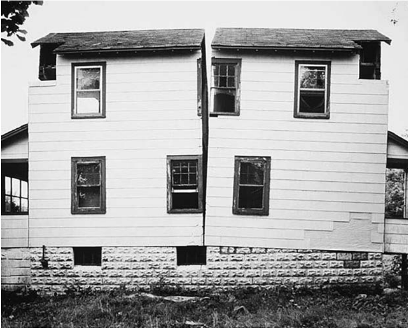
Figure 4.3 Gordon Matta-Clark's split house.
