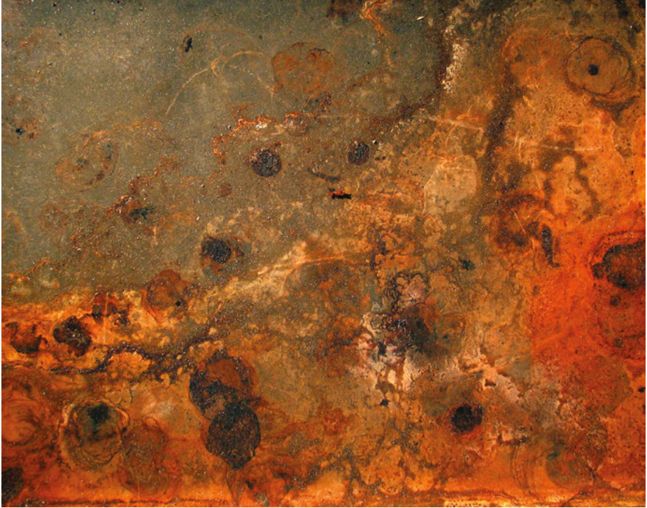
Fig. 4.10: Rust, the popular corrosion product of iron (Source: Roger McClassus 64 ).
