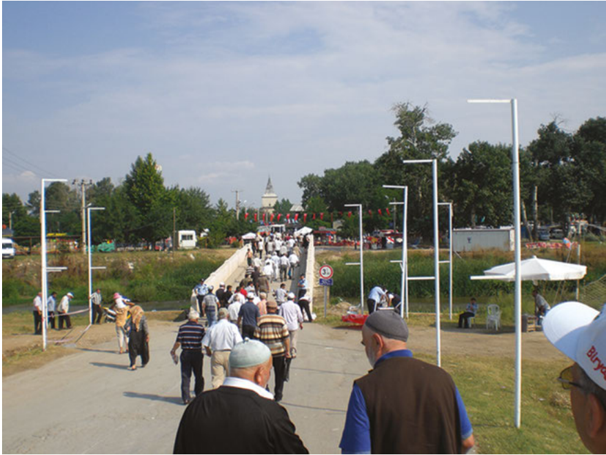
Fig. 19: Kanuni Bridge to Sarayıçi Island.
