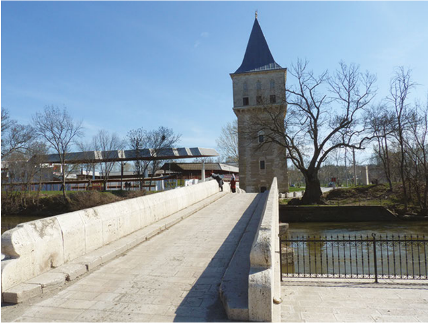
Fig. 20: Fatih Bridge from Tower of Justice and arena toward former Palace area.
