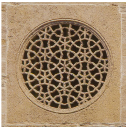
Fig. 7: Ekmekçioğlu Ahmed Paşa Caravanserai, detail of window grill eastern gable wall.
