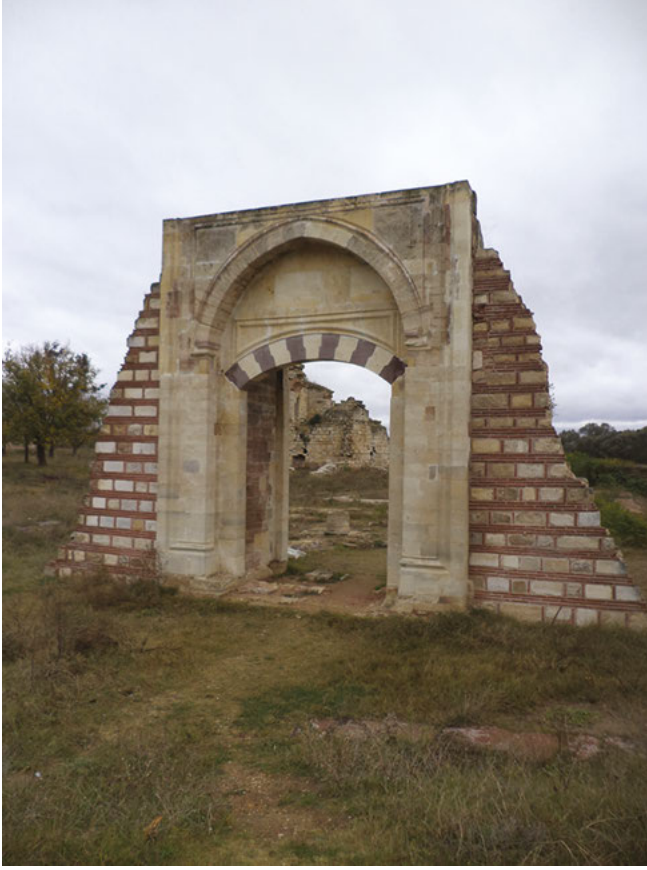
Fig. 3: Bab üs-Saade after the recent restoration.
