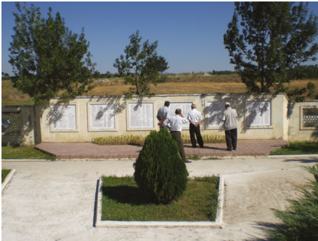
Fig. 11: Inner wall of BWMM III.
