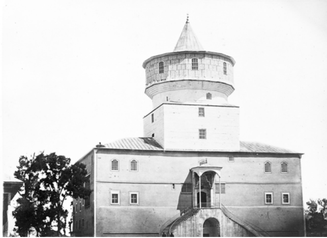
Fig. 1: The Belvedere after restoration.
