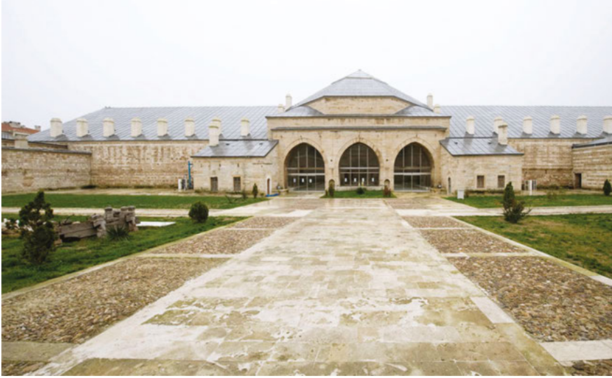
Fig. 8: Ekmekçioğlu Ahmed Paşa Caravanserai, courtyard.
