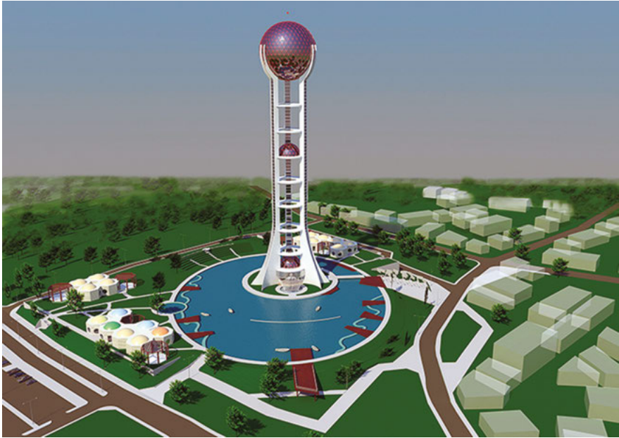
Fig. 9: The Edirne Sedef Kule tower project.
