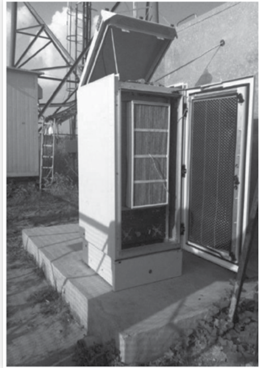
FIGURE B.3 Typical 5 kW stationary power fuel cell unit (source Intelligent Energy Ltd.: reproduced with permission).
