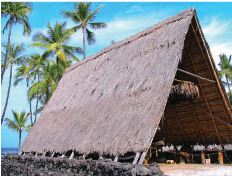
Hale were thatched externally most often with pili grass, but kō was used as an internal thatch to provide a finished look and sweet smell.
