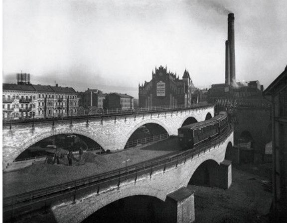
Viaduct of subway line (U2), Berlin, 1902. Photograph of the newly constructed train tracks that carved a new infrastructural space into the city near Gleisdreieck station.
