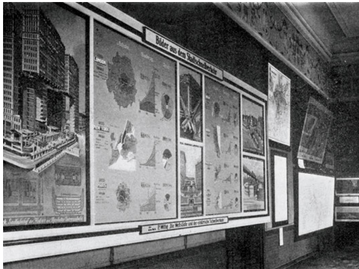
Display of comparative traffic diagrams of major cities at the Allgemeine Städtebau-Ausstellung , Berlin, 1910. The display title reads: “Images of high-speed city traffic.”
