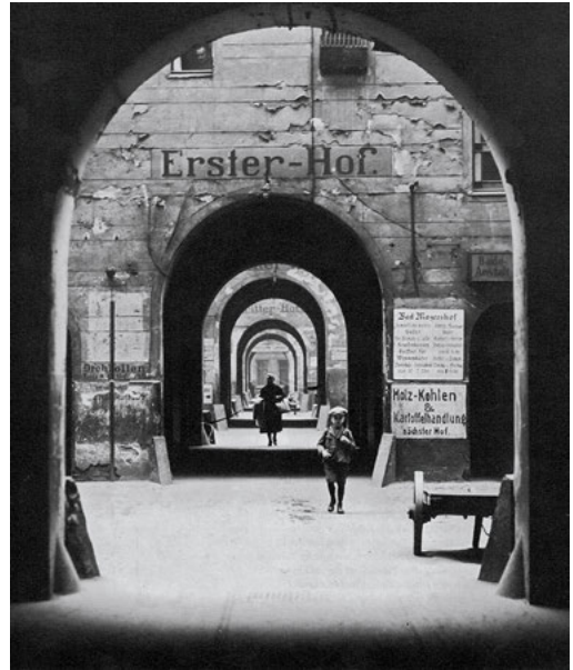
Meyer’s Hof, view from Ackerstraße 132/133, Berlin, c.1920. From the main entry along Ackerstraße, a clear view across all six courtyards opens up as each building volume doubles as a gate into the next courtyard.
