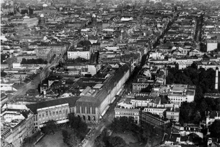
Aerial view of Leipziger Platz and Leipziger Straße, Berlin, c. 1930. The Warenhaus Wertheim is at the center of the photograph, with its façade along Leipziger Straße and turning the corner into Leipziger Platz.
