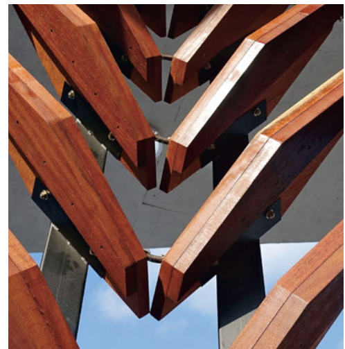
Element anchor and elastic connection
