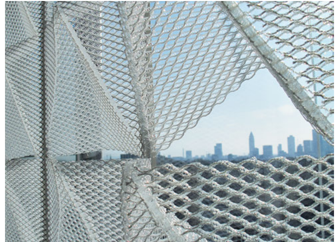
Pleated 3D textiles: hingeless opening mechanism with transparency control at the macro and meso levels
