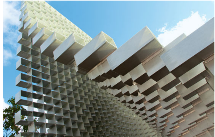
Fiberline's pultruded Lay Light profiles were used at the Serpentine Pavilion 2016, BIG (Bjarke Ingels Group), Kensington Gardens, London.
