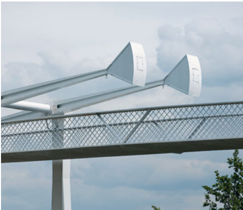
Counterweight (lever arm)
