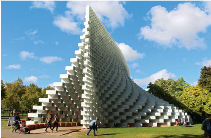
Fiberline's pultruded Lay Light profiles were used at the Serpentine Pavilion 2016, BIG (Bjarke Ingels Group), Kensington Gardens, London.
