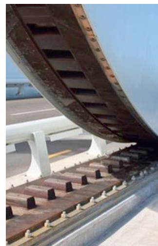
Underside of bridge arm and rack
