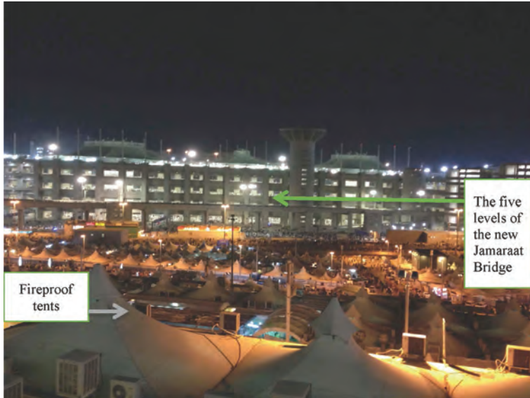
Fig. 13.3: The new Jamaraat Bridge and fireproof tents (photo credit: Jahanzeeb Qurashi).
