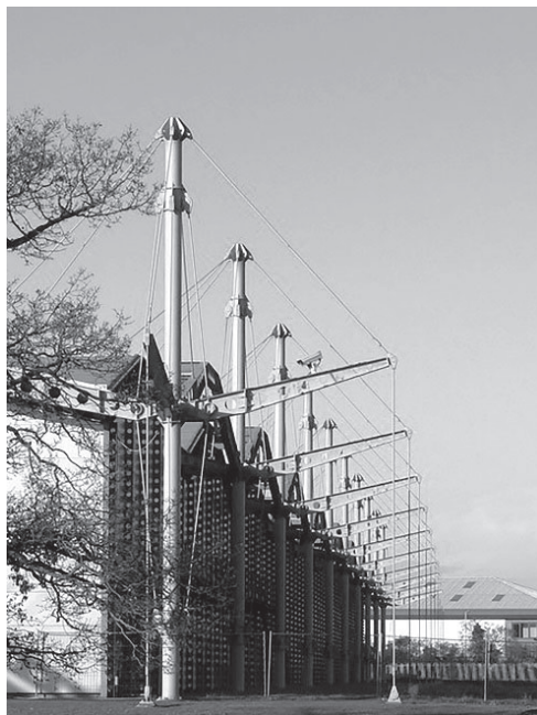
14. Renault Centre, Swindon, England, Norman Foster, 1982. Architecture based on the principle that the latest developments in science and technology should represent the modern era.
