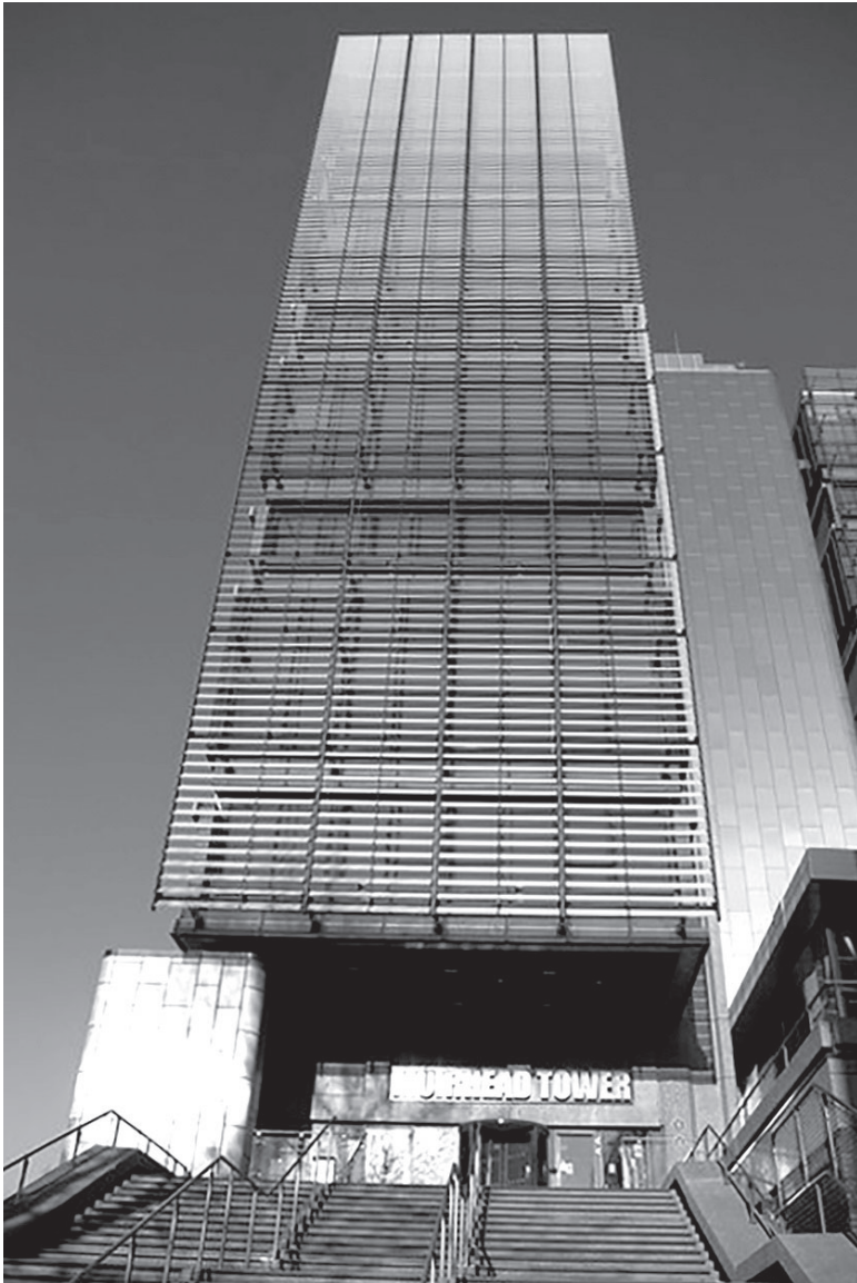
15. Muirhead Tower, University of Birmingham, England. Due to be demolished after expensive refurbishment. The short investment cycle of new buildings does not encourage the use of enduring materials.
