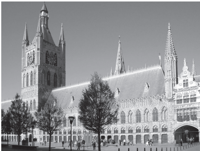
15. Ypres Cloth Hall, Ypres, Belgium, completed 1304 CE and destroyed in the 1914-18 War. Reconstructed in its original form from 1933 to 1967.
