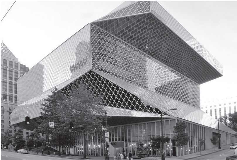
14. Seattle Public Library, Seattle, Washington State, USA, Rem Koolhaas, 2004. The idea of newness and difference carries with it a sense of exhilaration.
