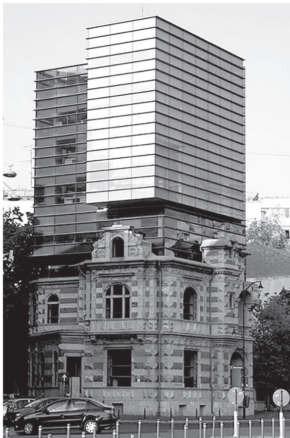
17. Romanian Architects' Union Building, Bucharest, Romania, Dan Marin, Zeno Bogdnescu, 2007. The preservation of historic buildings is supported by modernist architects as it can demonstrate the contrast between the past and present and the 'authenticity' of difference.
