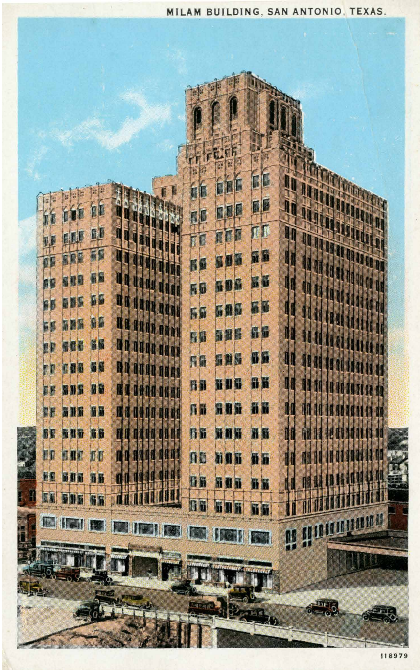
Figure 2. Milam Building, San Antonio, TX, 1925. George Willis was the architect and Willis Carrier oversaw the design and installation of the air conditioning system. (Credit: Author's collection.)
