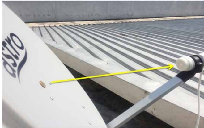
Figure 8. The reflection of the coin can be visualized at the feed
