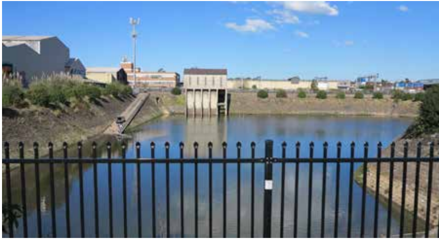
Figure 15.3. Sydenham Stormwater Drainage Pit and Pumping Station.
