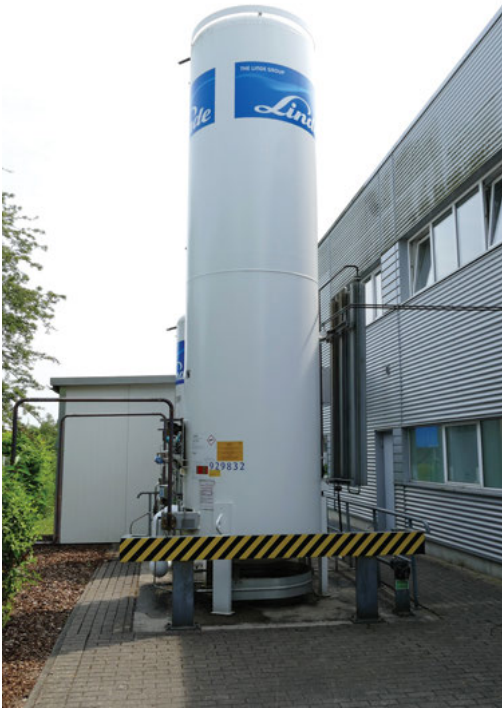
Figure 3.46: Tank for liquid argon. Printed with the friendly permission of SPECTRO Analytical Instruments GmbH, Boschstr. 10, 47533 Kleve, Germany.
