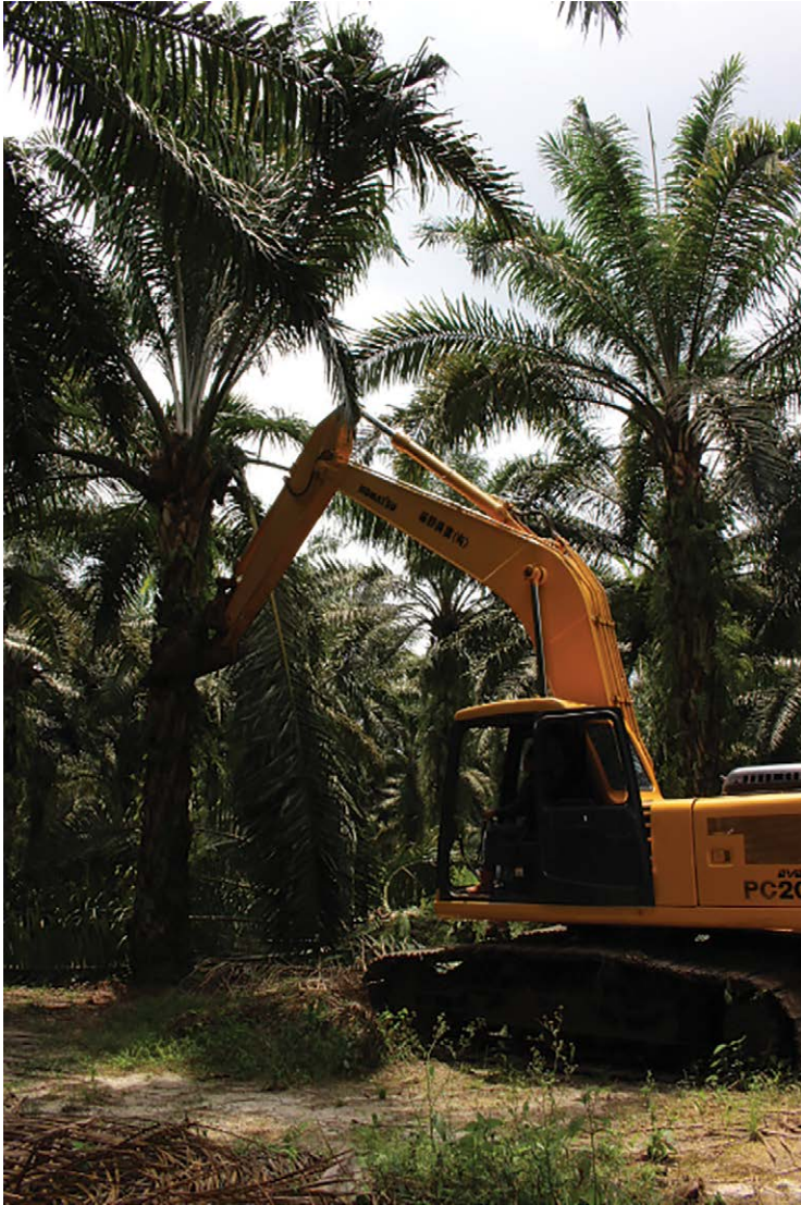
Fig. 4.7. Tractor pushing over an oil palm tree.
