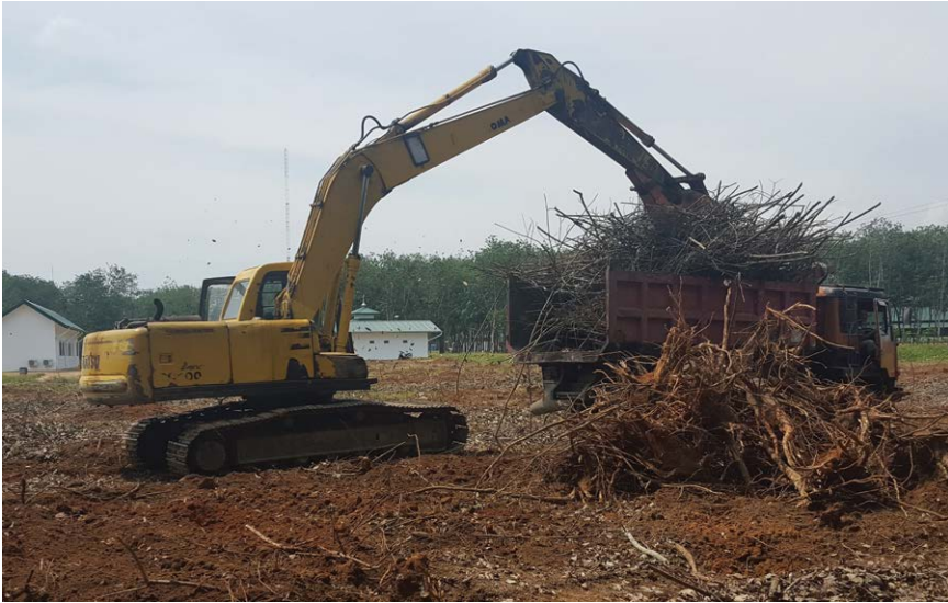
Fig. 4.2. All rubber roots and small branches are allowed to dry, and then removed and gathered outside the plantation.
