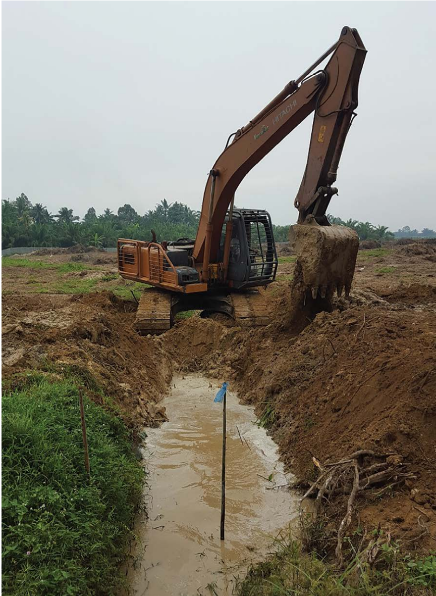
Fig. 6.2. Making a drain using heavy machinery.
