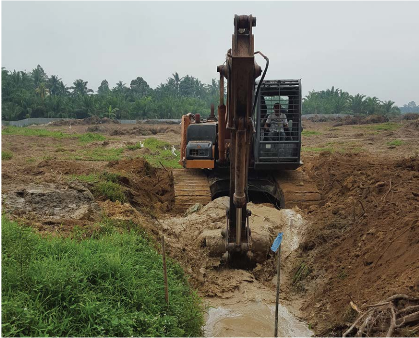
Fig. 4.3. Excavation of a drain with heavy machinery.
