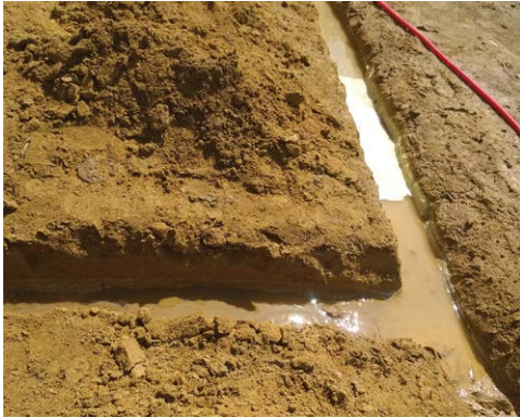
Fig. 3.2. Nursery drainage canal (typically 30 cm for width and 50 cm for depth).
