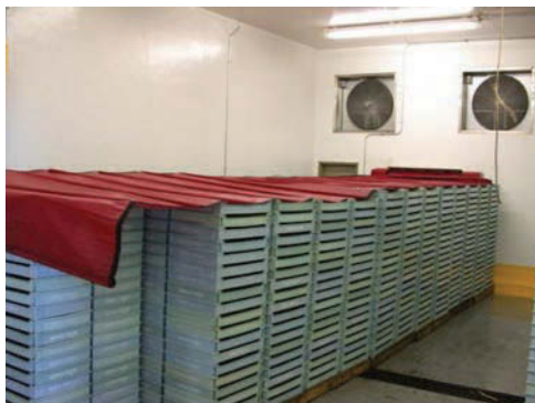
Fig. 15.8. Pallettes of blackberries placed for forced air cooling using a false wall plenum for pushing out air (P. Perkins-Veazie).
