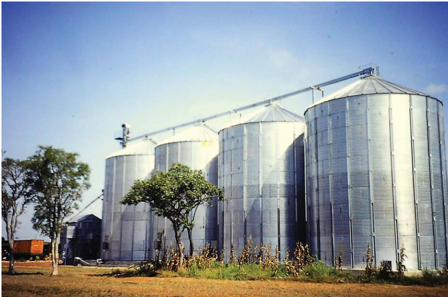
Fig. 6.3. Large modern silo in which grain can be protected by fumigation.
