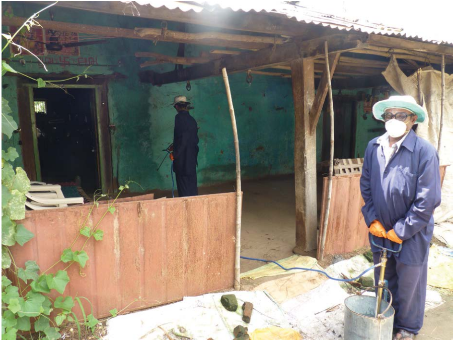
Fig. 9.18. Vector control in India using a stirrup pump and a second person with a lance inside the house to apply an indoor residual spray.
